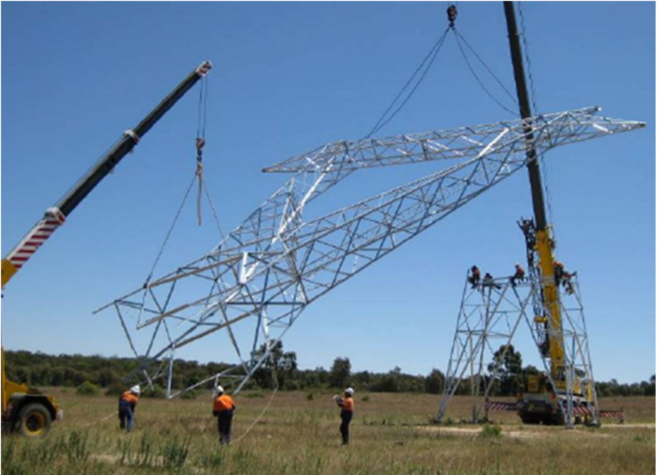
Photo A-1 Structure assembly using cranes
