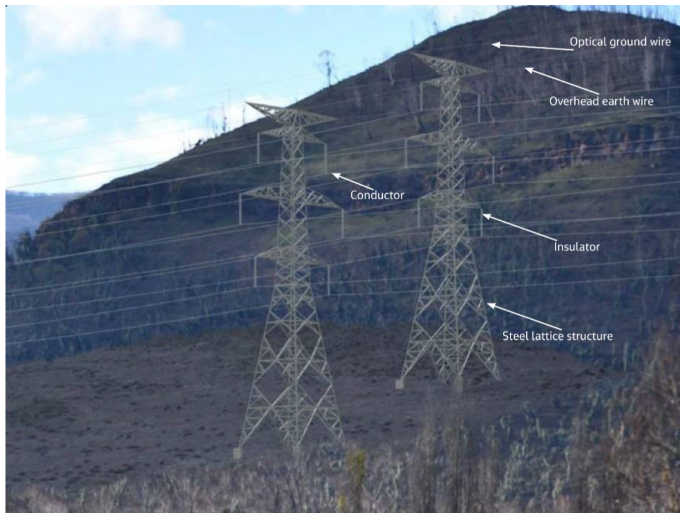
Figure 5-2 Indicative concept design for the transmission structures
