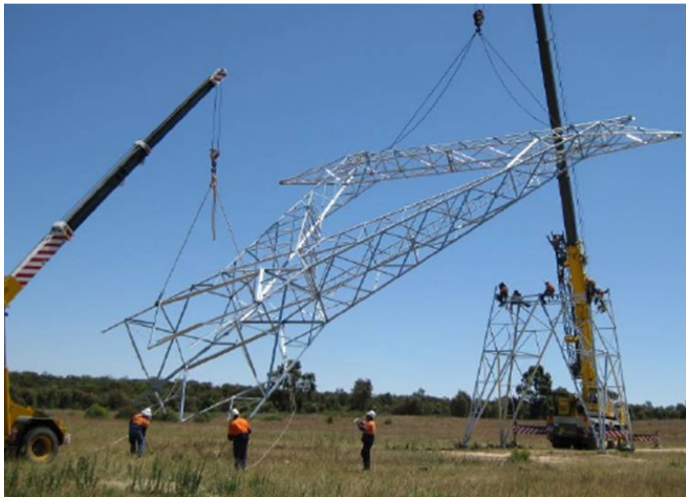
Photo 5-1 Structure assembly using cranes
