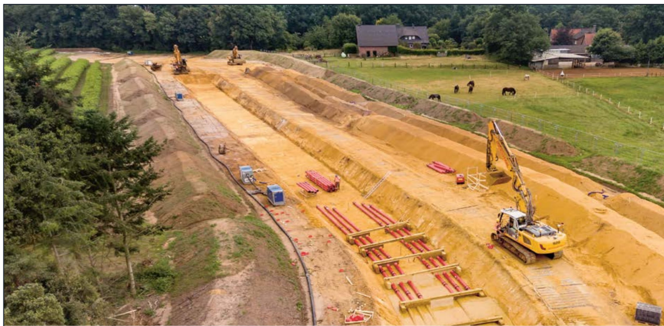
Photo 3-1 Example of a trenched double circuit underground transmission connection
