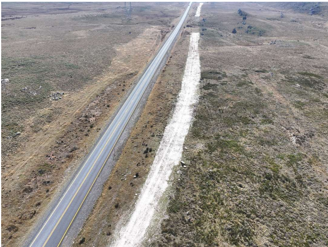
Chainage 1800 – 2300 (Gooandra Trail site entrance laydown) (SMH section) (L1)
