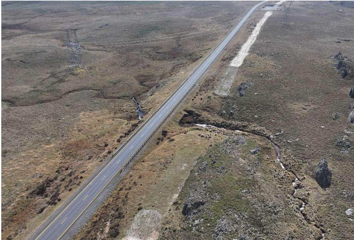
Chainage 1500 Powerline Creek - 1800 (SMH section)
