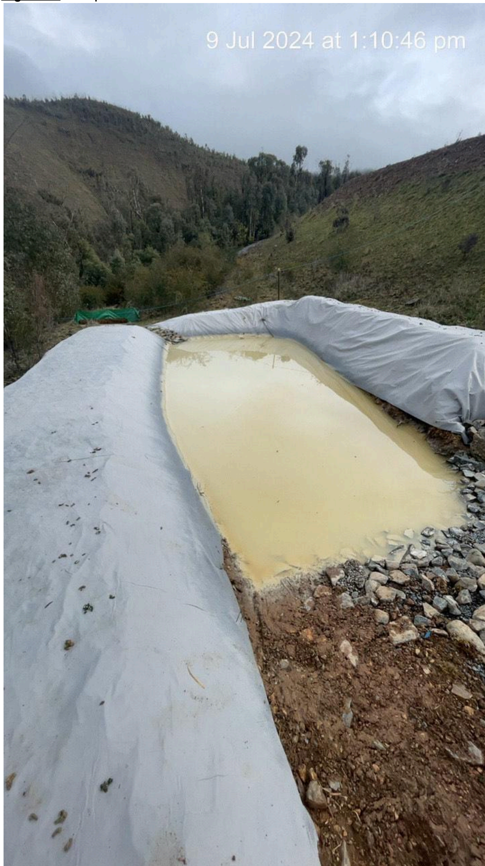
Figure 2: Sump A at the time of the incident.
