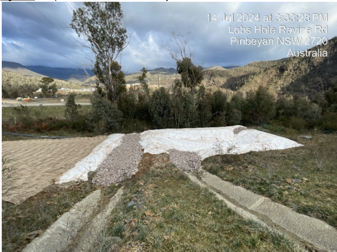
Figure 6: Sump A after rectification works by LEED contractor.
