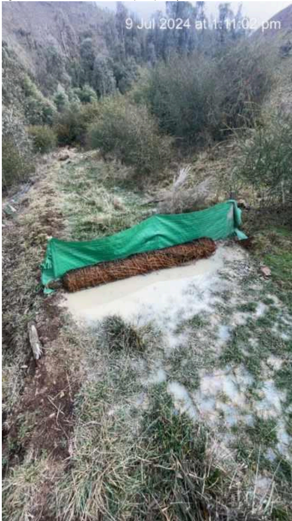
Figure 3: Downstream of the Sump A spillway
