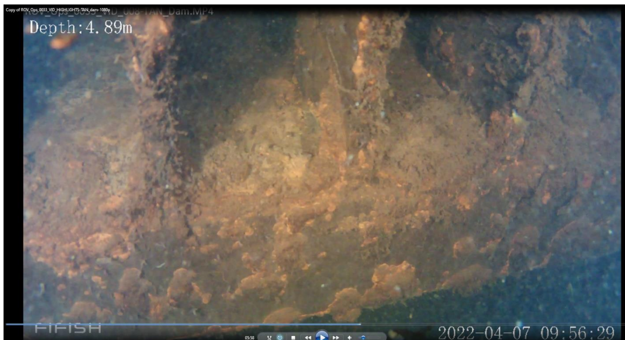
Figure 10: Example of biofouling accumulating on the surface of the existing Tantangara ROW coarse screens
