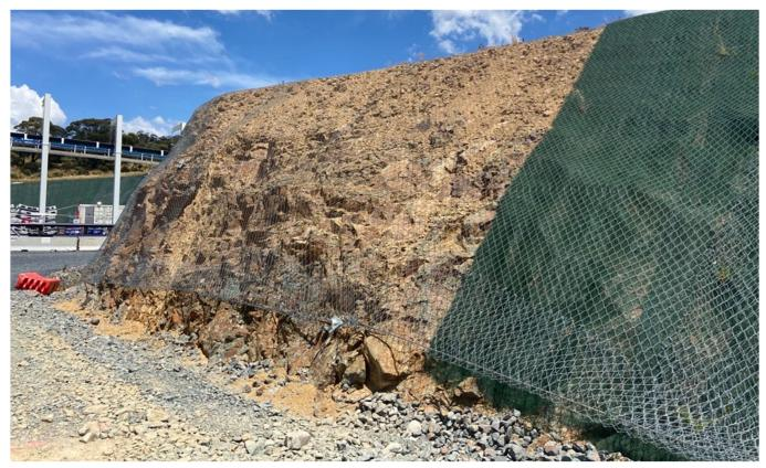
Figure 3.2 Cutting at Tantangara Adit portal in moderately weathered rhyodacite.
