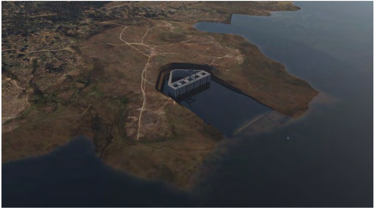
Figure 3: Artist impression of Tantangara Reservoir at MOL showing the excavation and concept design of the SWIFF drum structure. The boat just out of the intake channel is 6.7m long.
