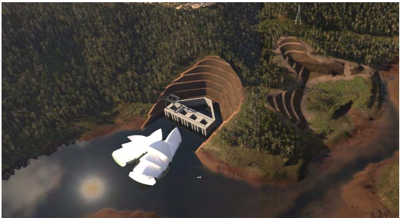
Figure 4: Artist impression of Talbingo Reservoir at MOL showing the excavation and concept design of the SWIFF drum structure. The boat just out of the intake channel is 6.7m long. The Sydney Opera house is also included to provide an additional indication of scale.
