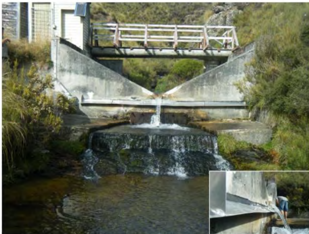
Figure 5. Example of a v-notch built barrier from New Zealand, with a horizontal metal angle ‘lip barrier’ to prevent fish climbing up the wall.
