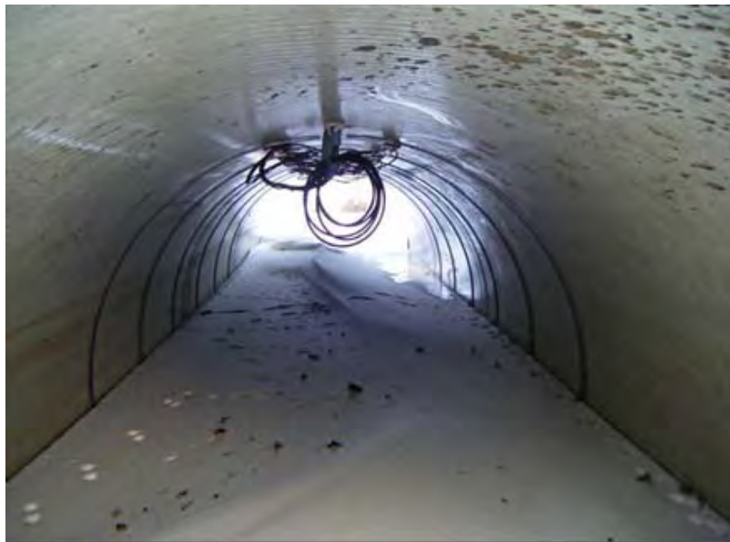
Figure 27 Example of culvert electrical barrier at lake outlet. White Lake, Minnesota, USA (Smith-Root).
