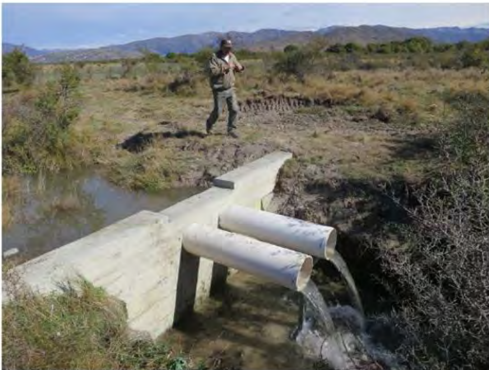
Figure 4. An example of a built barrier in NZ with pipe extensions to remove wetted climbing pathways during low flow.
