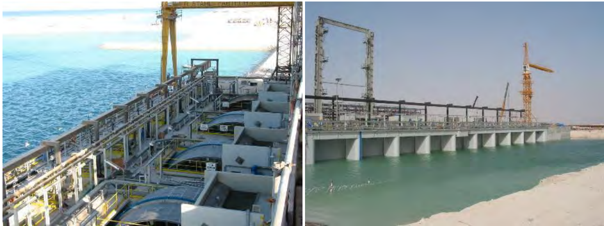
Figure 13 Drum screen screening installation at Ras Laffan Common Cooling Water Intake, Qatar. 14 drum screens are installed with a combined flow capacity of 333 \text{ m}^3 \text{ s}^{-1} (courtesy of Ovivo).
