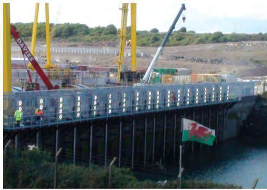
Figure 21 FGS Synchronised Intense Light and Sound (SILAS) sound projectors raised for inspection at Pembroke Power Station, UK. LED lights can be seen illuminated (courtesy FGS Ltd).
