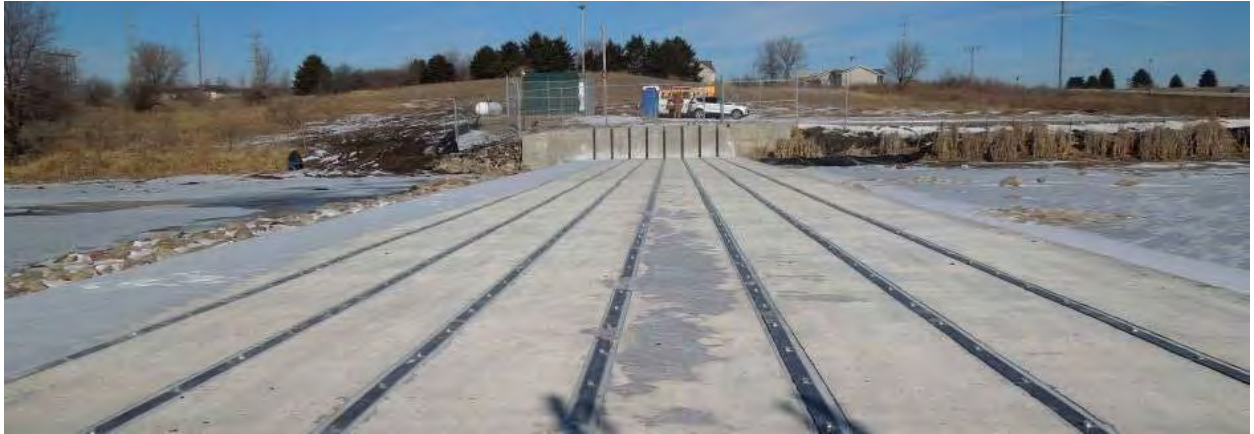
Figure 26 Example of bottom-mounted, open channel electrical barrier in channel with water drawn down. Okoboji Lake outlet in Iowa, USA (Smith-Root).
