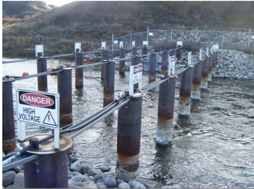
Figure 28 Example of vertical electrode barrier system at power plant tailrace to prevent the movement of fish upstream into the tailrace. Battle River Generating Station, Alberta, Canada (Smith-Root).
