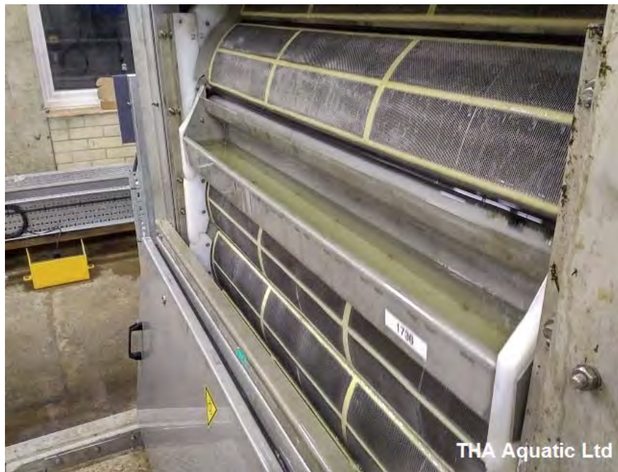
Figure 15 Fish buckets fitted to a dual-flow band screen (photo THA Aquatic Ltd).
