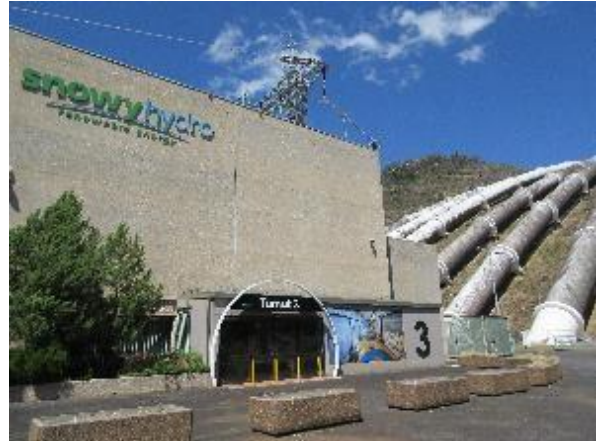
Figure 53 Tumut 3 Power Station
