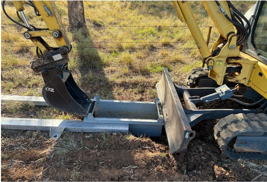
Figure 5: Sampling frame placed into access trench between the guide sleepers.
