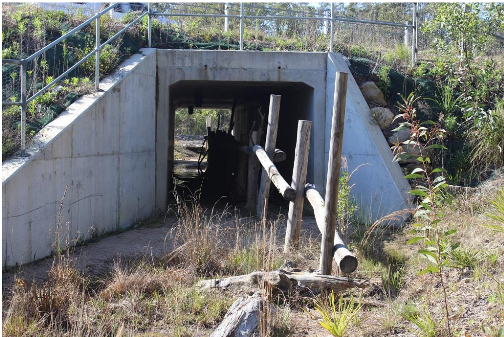
Photo 1 Dedicated Koala culvert with fauna furniture under the Pacific Highway at Glenugie
