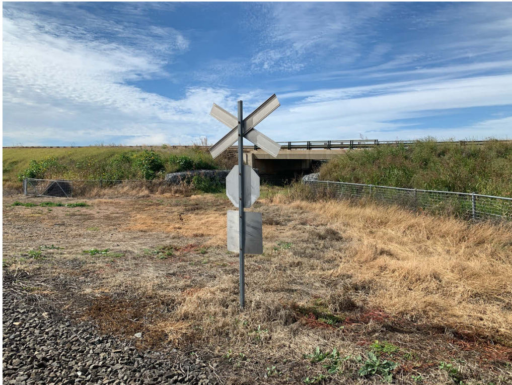
Appendix 4: View of the approach to existing underpass under the Newell Highway from the shunt railway track. Note that fencing in this section is mostly sound, with the exception of light wire gates at entry points.
