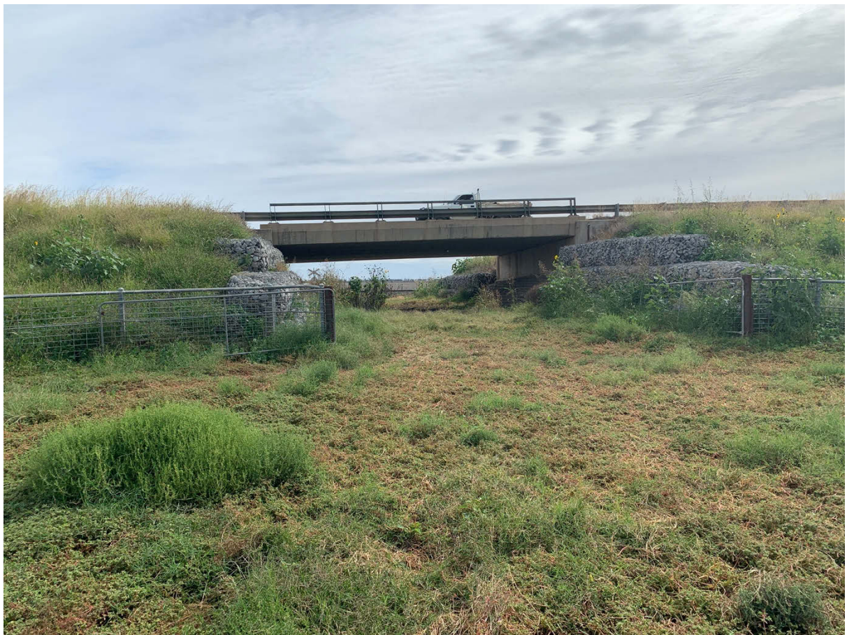
Figure 1-3: Current stock underpass under the Newell highway (Orientation: West)
