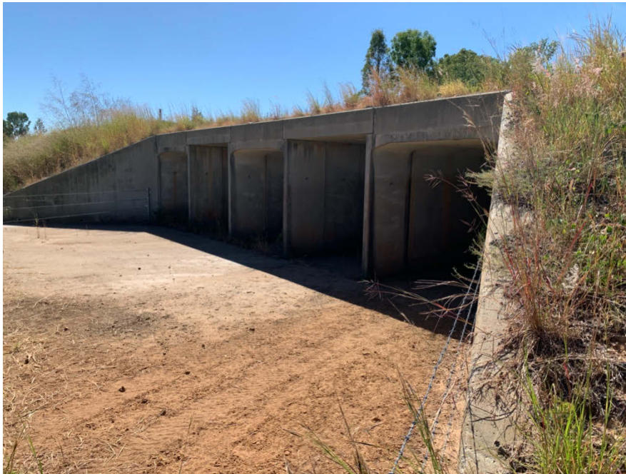
Figure 3-2: A cattle underpass/causeway (Carnarvon Highway, QLD) demonstrating what to avoid in building wide underpasses with multiple culverts. Cattle flow is difficult to maintain unless animals are well trained. Note use of wing walls funnels animal attention and movement towards the culvert.
