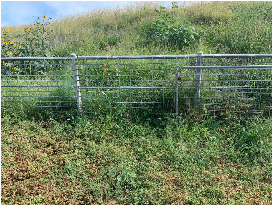
Appendix 6: Fencing type on eastern side of existing underpass. Holding pen on this side of underpass is in good condition.
