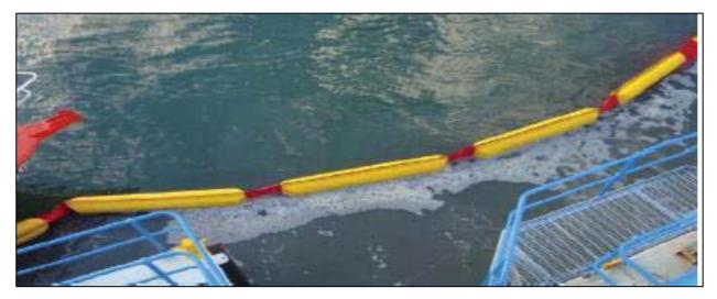
Figure 5 Silt Curtain to deployed around dredging and disposal works areas
