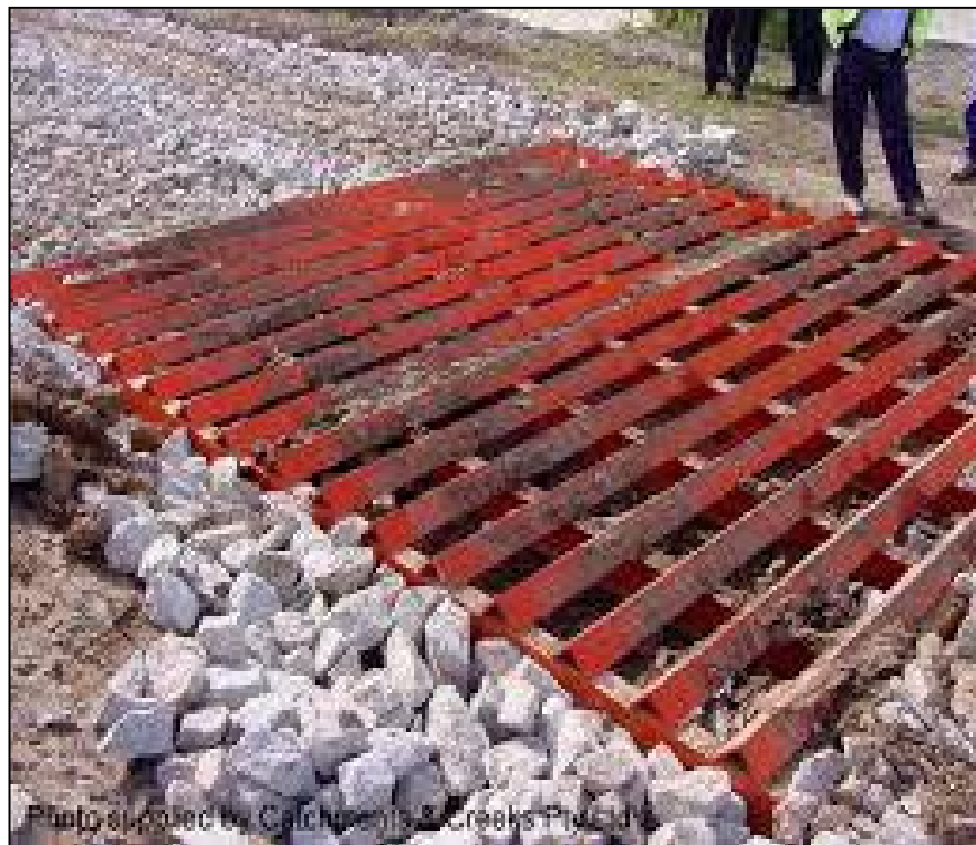
Figure 6.1 Rumble grid to be installed at MBD Site Compound and Emplacement Cell Construction Sites
