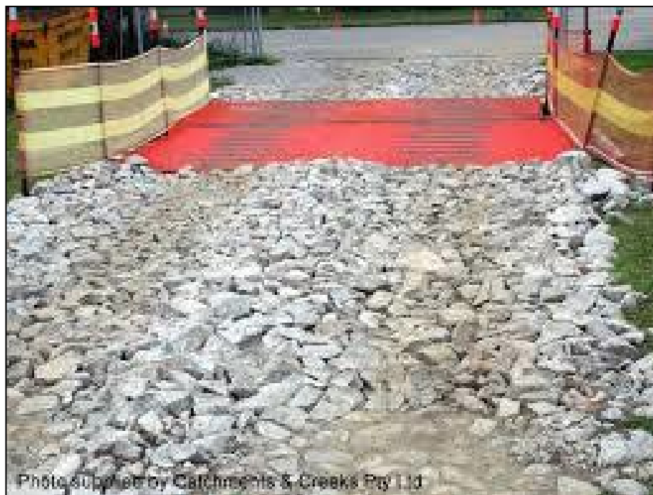
Figure 6.2 Gravel haul road to be installed at MBD Site Compound and Emplacement Cell Construction Sites
