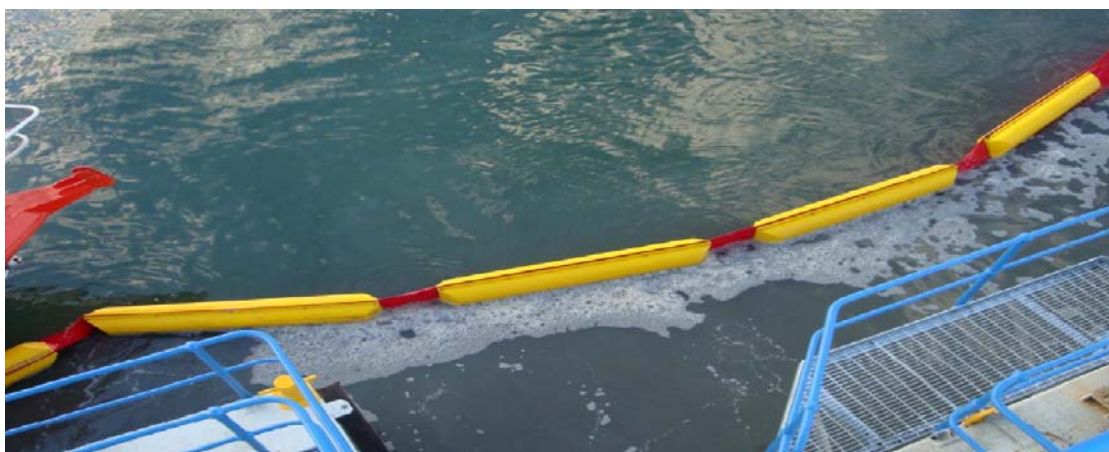
Figure 12-7 Example of a silt curtain surrounding a dredging operation
