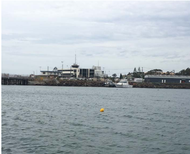
Photograph 2 Wharf at east end of reclamation area (03/10/2018)
