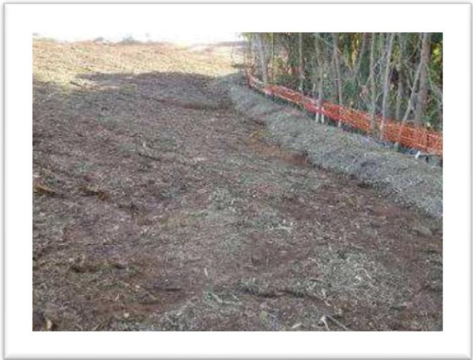
Figure 9 Example of mulch berm
