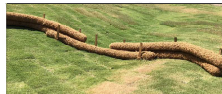
COIR LOG SEDIMENT TRAP (FOR INSTREAM)
