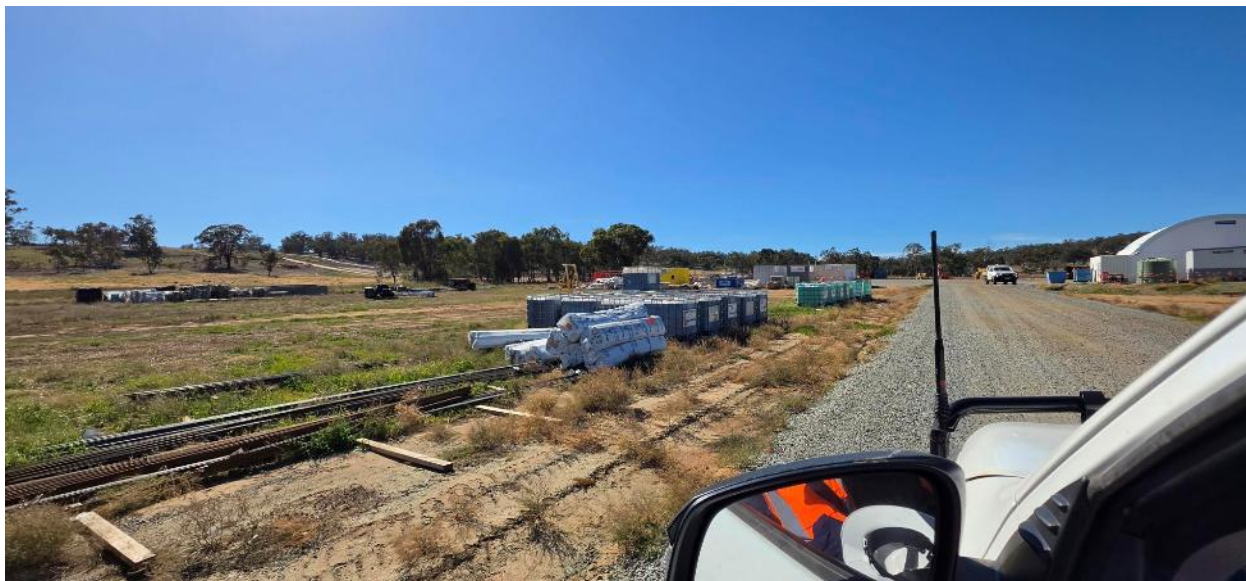
Polymer available on site for stabilisation and dust suppression.
