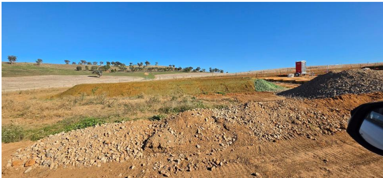
Stockpiled material to be crushed and reused for cut and fill works.
