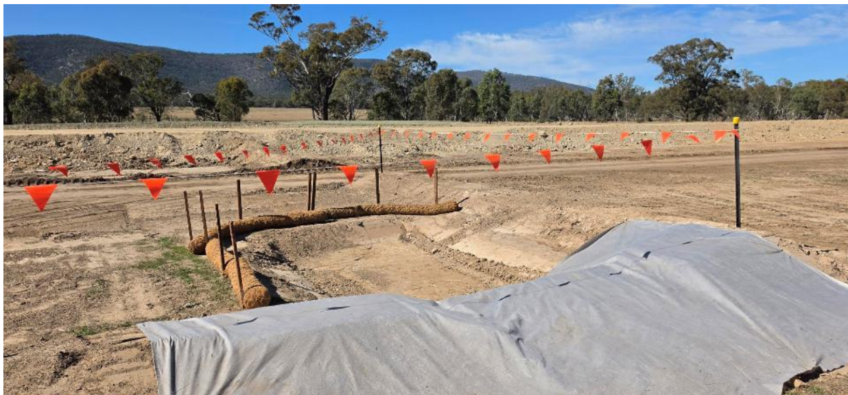
Excavated sediment trap along the alignment.
