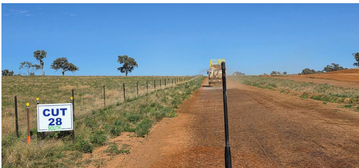
Water cart actively operating along the access alignment for dust suppression.
