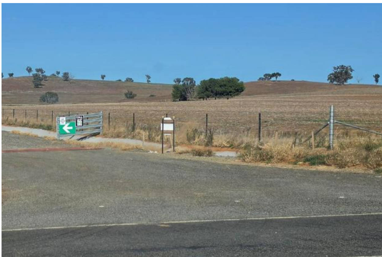
Rumble Grid in place at Gate 7A to control mud tracking.
