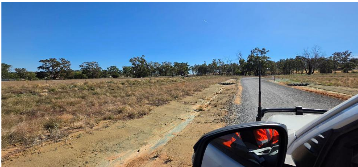
Rock checks in place along the swale drain at Dirnaseer Compound.
