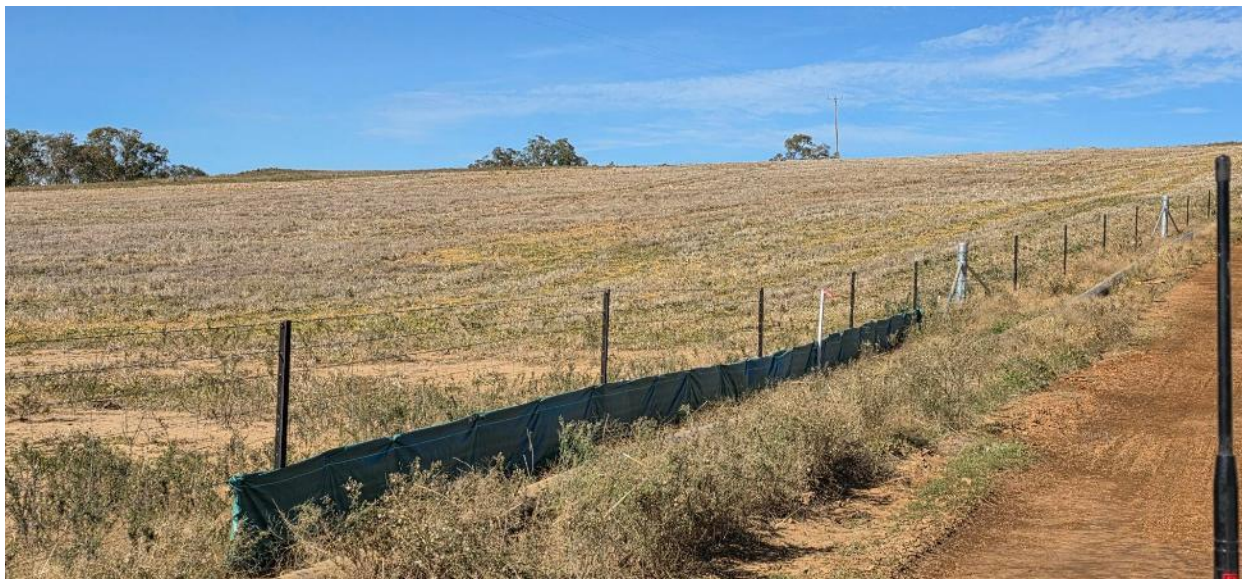
Sediment fences installed and observed at low points along the alignment.
