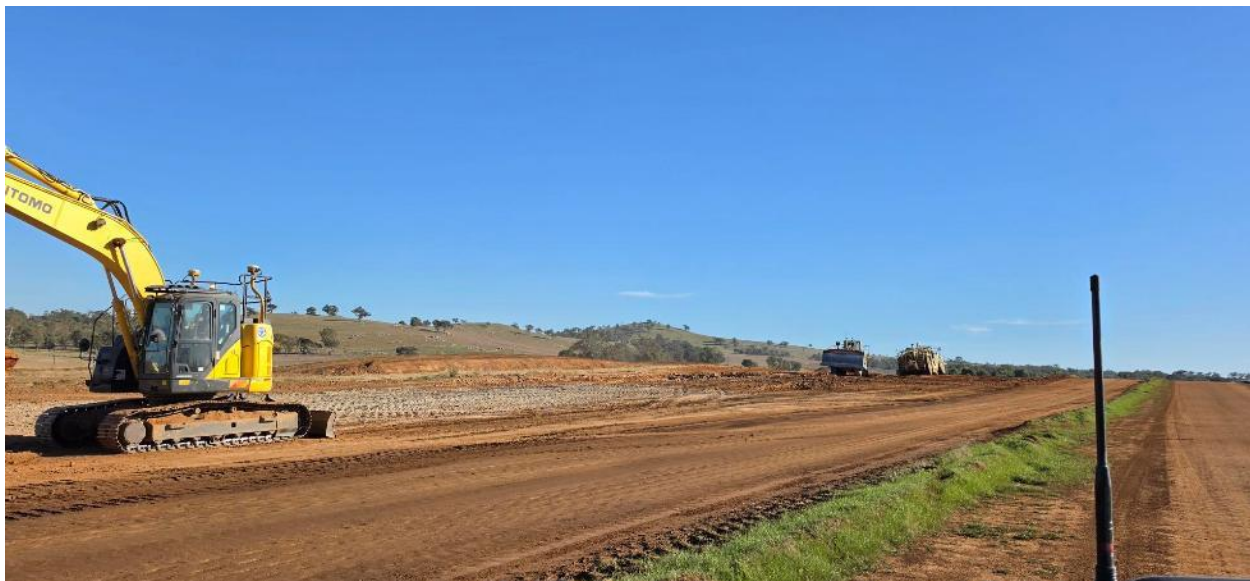
Earthworks in progress along the alignment – no dust observed.
