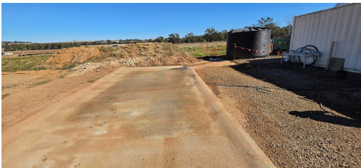
Vehicle washdown area at Dirnaseer Compound.
