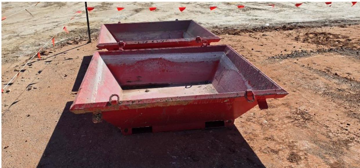
Concrete washout trays.
