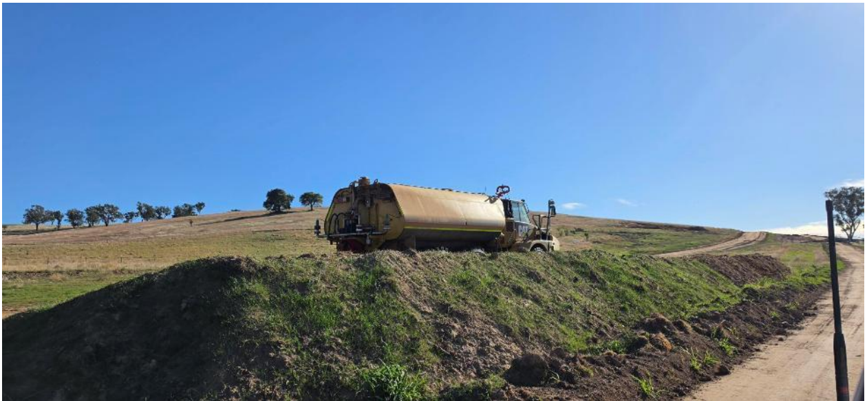
Water cart available on site.
