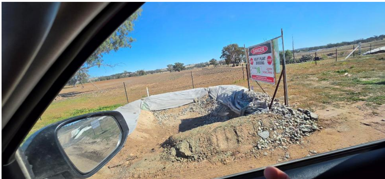
Excavated sediment trap installed along the alignment.
