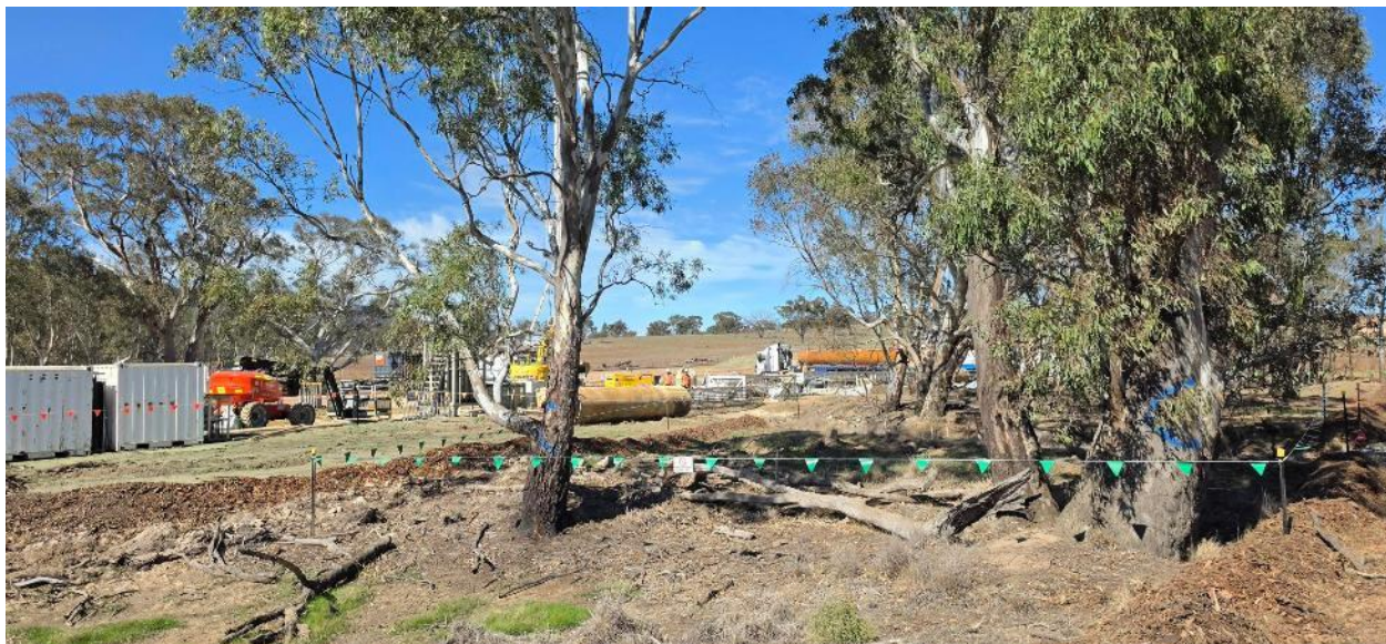
Green flagging installed for habitat trees at Run Boundary Creek.
