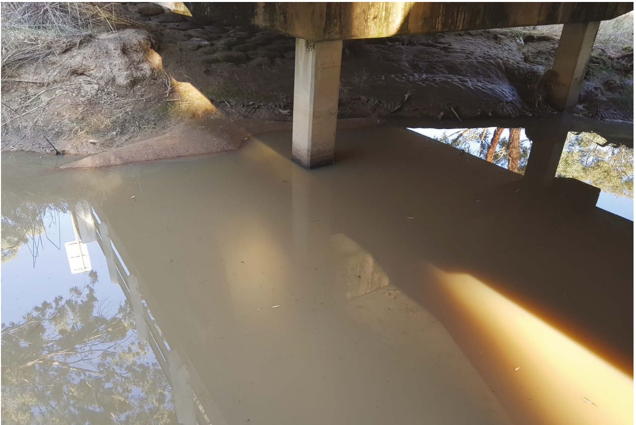
PHOTO 13-4: PHOTO OF DUDAUMAN CREEK LOOKING UPSTREAM UNDER THE ROAD BRIDGE DURING APRIL 2021 SAMPLING EVENT
