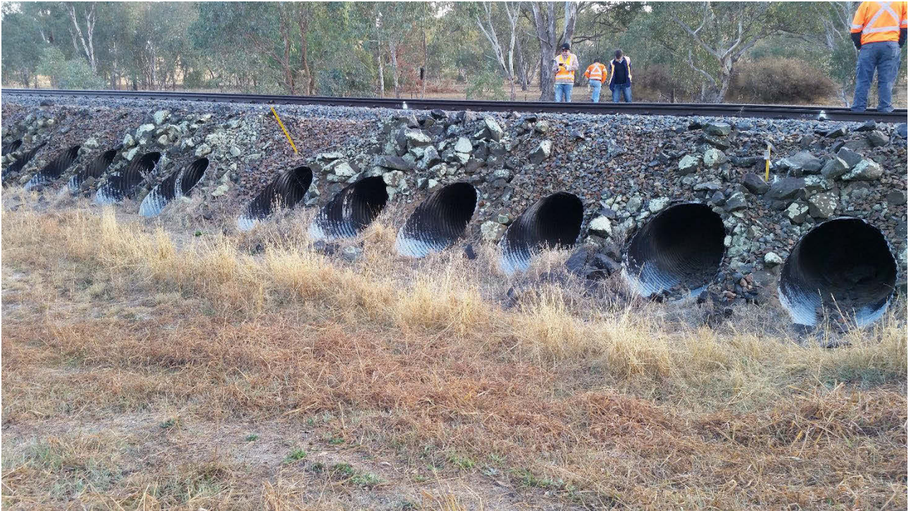
Photo 6.6 Eastern Culvert bank under Lake Cargelligo line
