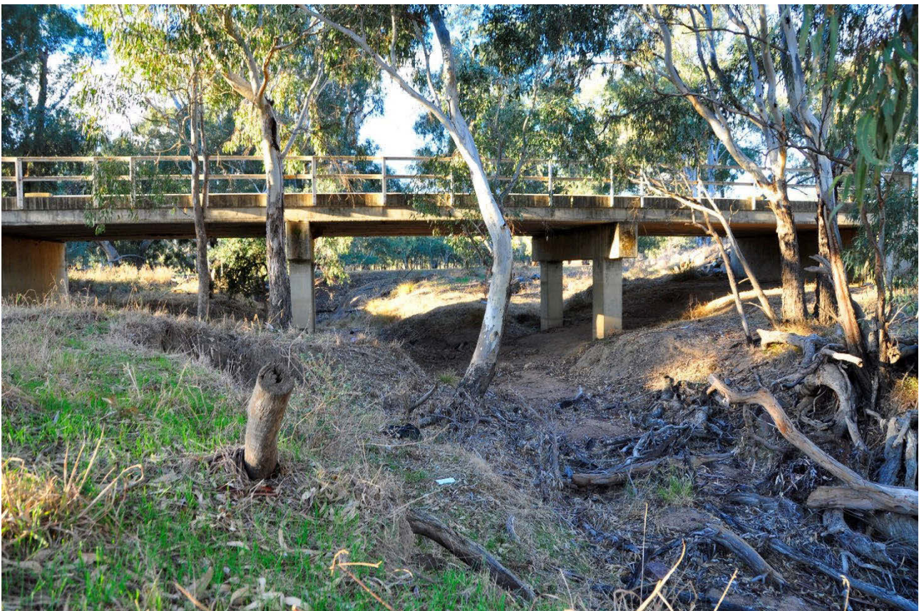
Photo 6.11 Ironbong Road bridge across Ulandra Creek, looking upstream
