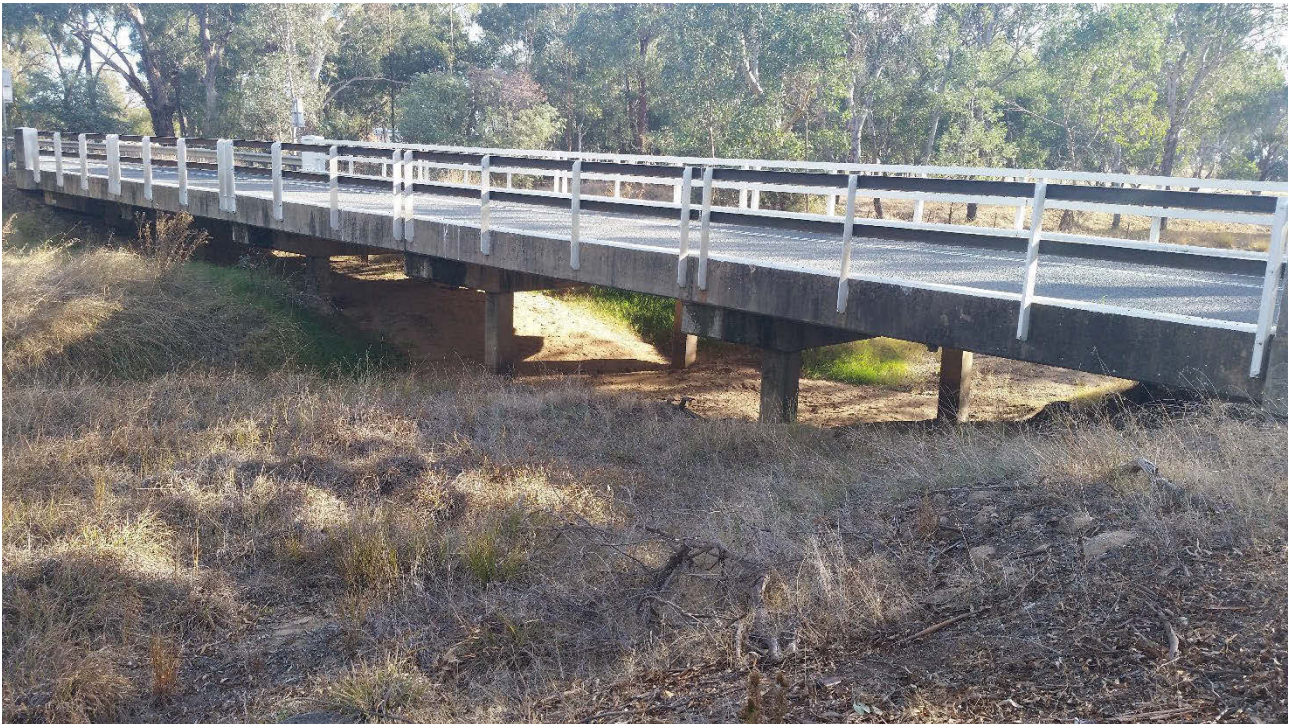
Photo 6.3 Burley Griffin Way Eastern Crossing looking downstream
