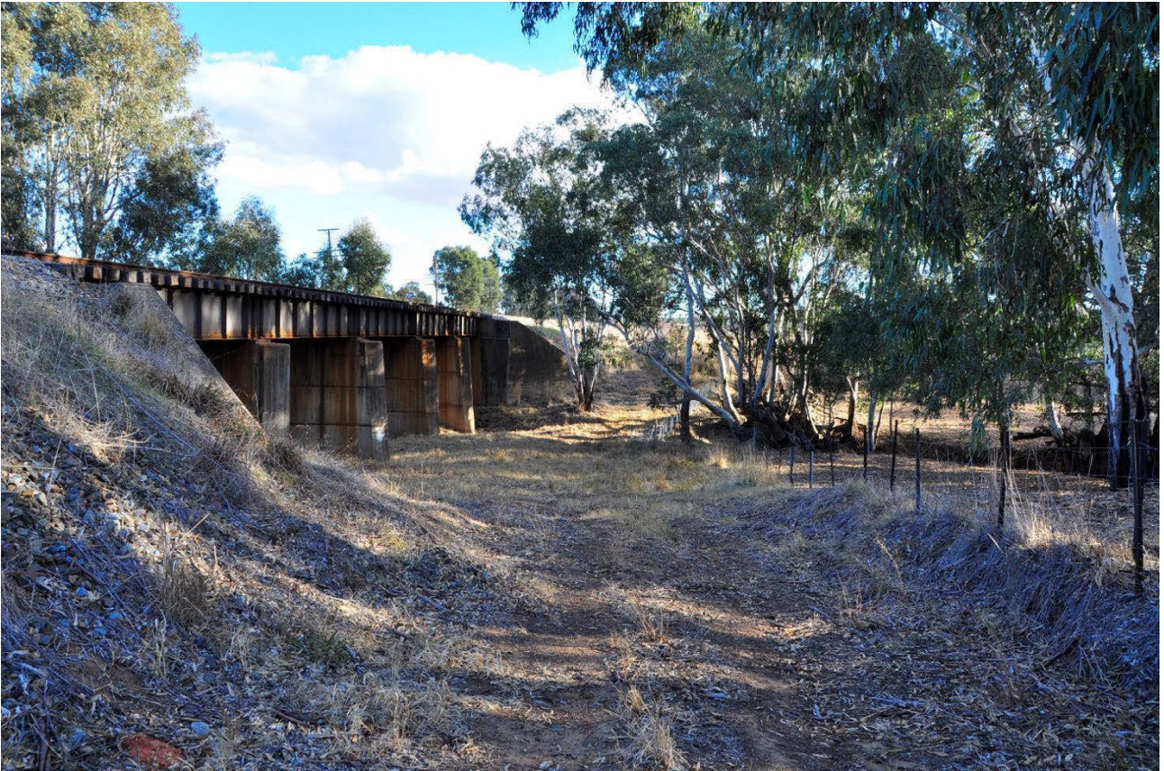
Photo 6.9 Billabong Creek rail bridge upstream, left bank
