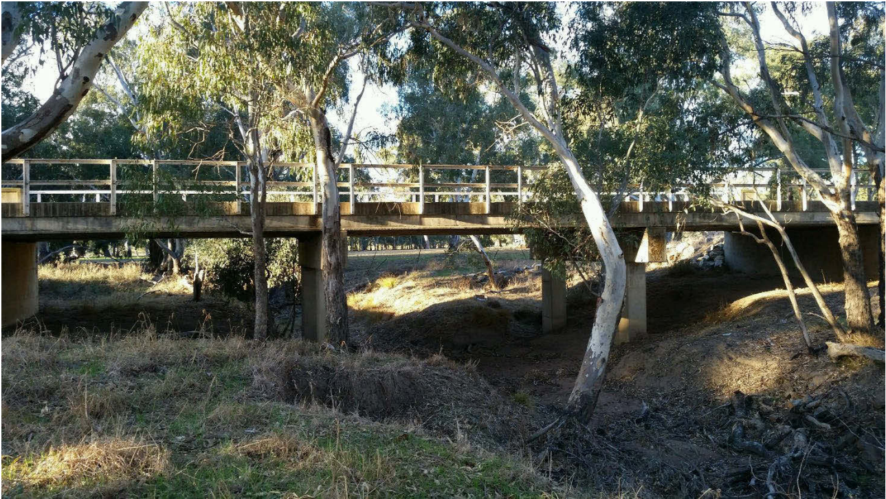
Photo 6.1 Ulandra Creek bridge at Ironbong Road
