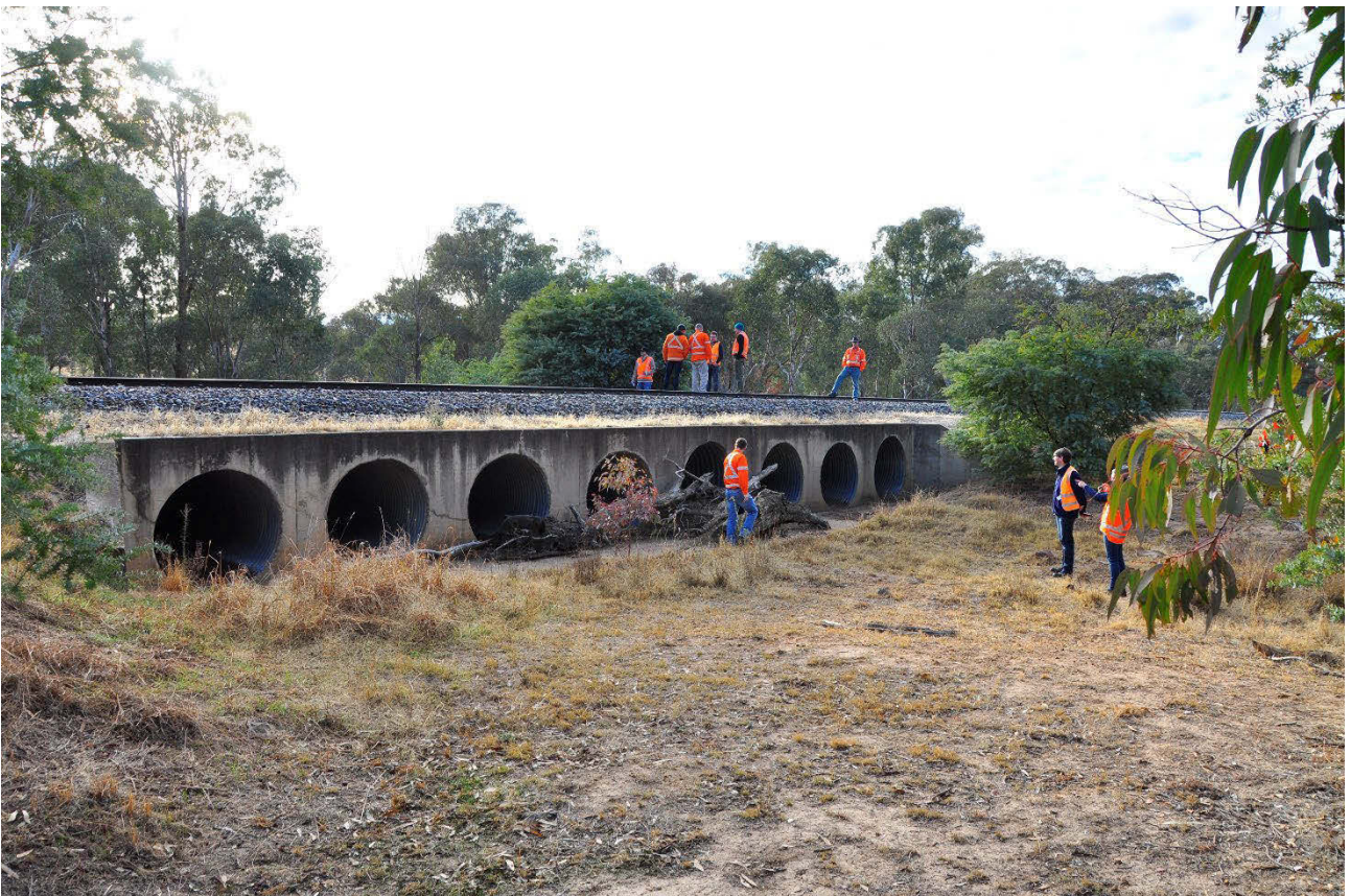
Photo 6.5 Lake Cargelligo Rail line western crossing of Dudauman Creek
