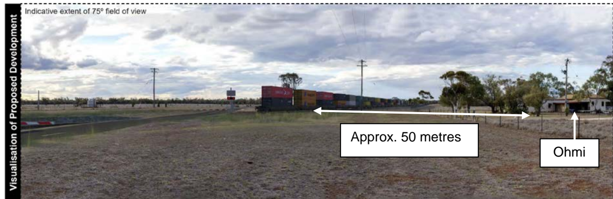
Figure 11 | visual impression of the level crossing near ‘Ohmi’ residence 254050 (Source EIS)
