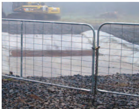
FIGURE 7.8: Wheel wash bay used at Sassafras during upgrades on Main Road 92 (Nowra to Nerriga) Southern Region. Vehicles drive onto the grid and are washed down. Water is contained under the grid (Photo: Julian Watson).
