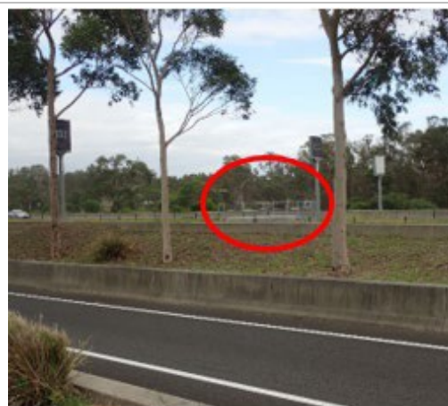
Tunnel Shaft 4 as viewed from eastern road reserve, facing southwest
