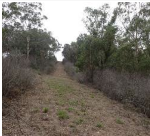
View of surface over northeast section of the pipeline, facing northeast
