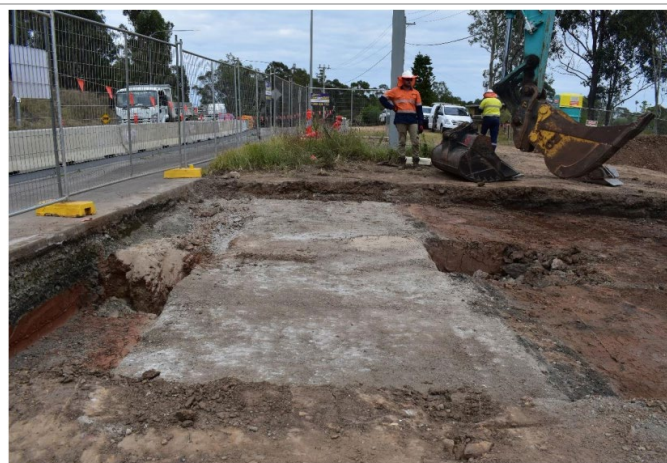
Non-significant concrete slab remains found during monitoring undertaken for the M12 Motorway project
