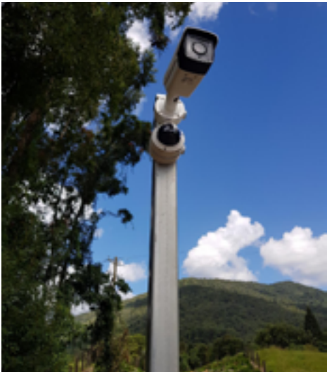
CCTV pole mounted camera
