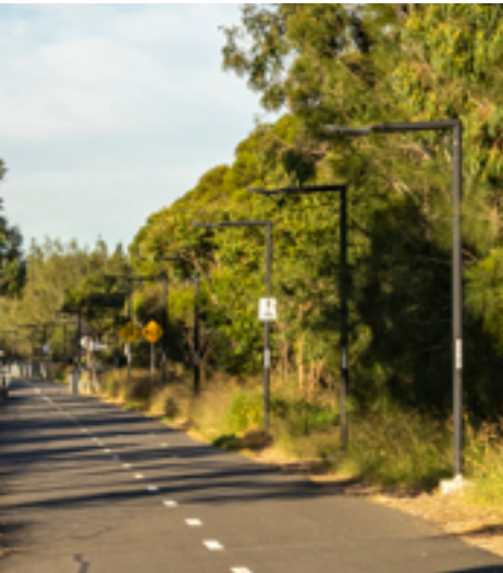
Typical M7 shared path lighting element
