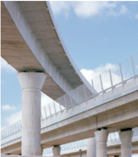
Box girder - M7 Motorway
