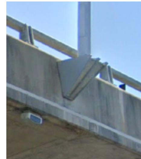
Existing M7 Motorway lighting corbel
