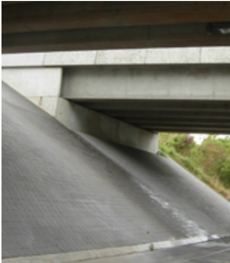
Spill through abutment
