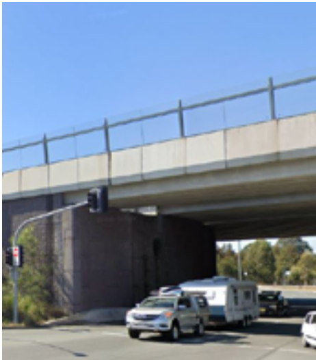
Walled abutment - Banora Point Upgrade
