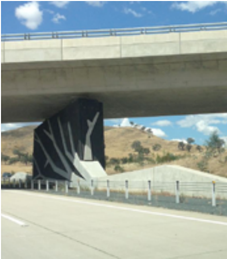
Voided slab - Wagga Wagga overpass
