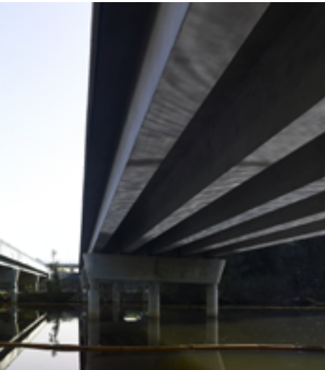
Super-T girder - Bonville Bypass
