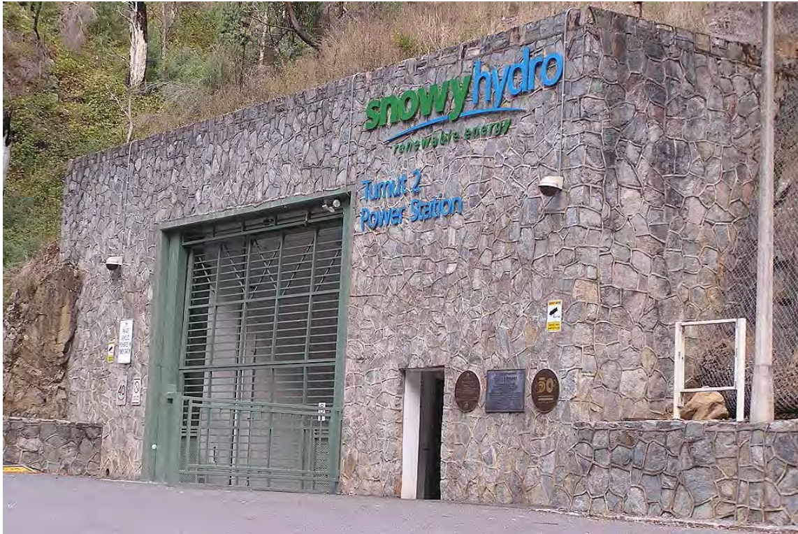
Photograph 7.1 Finished Tumut 2 power station tunnel portal
