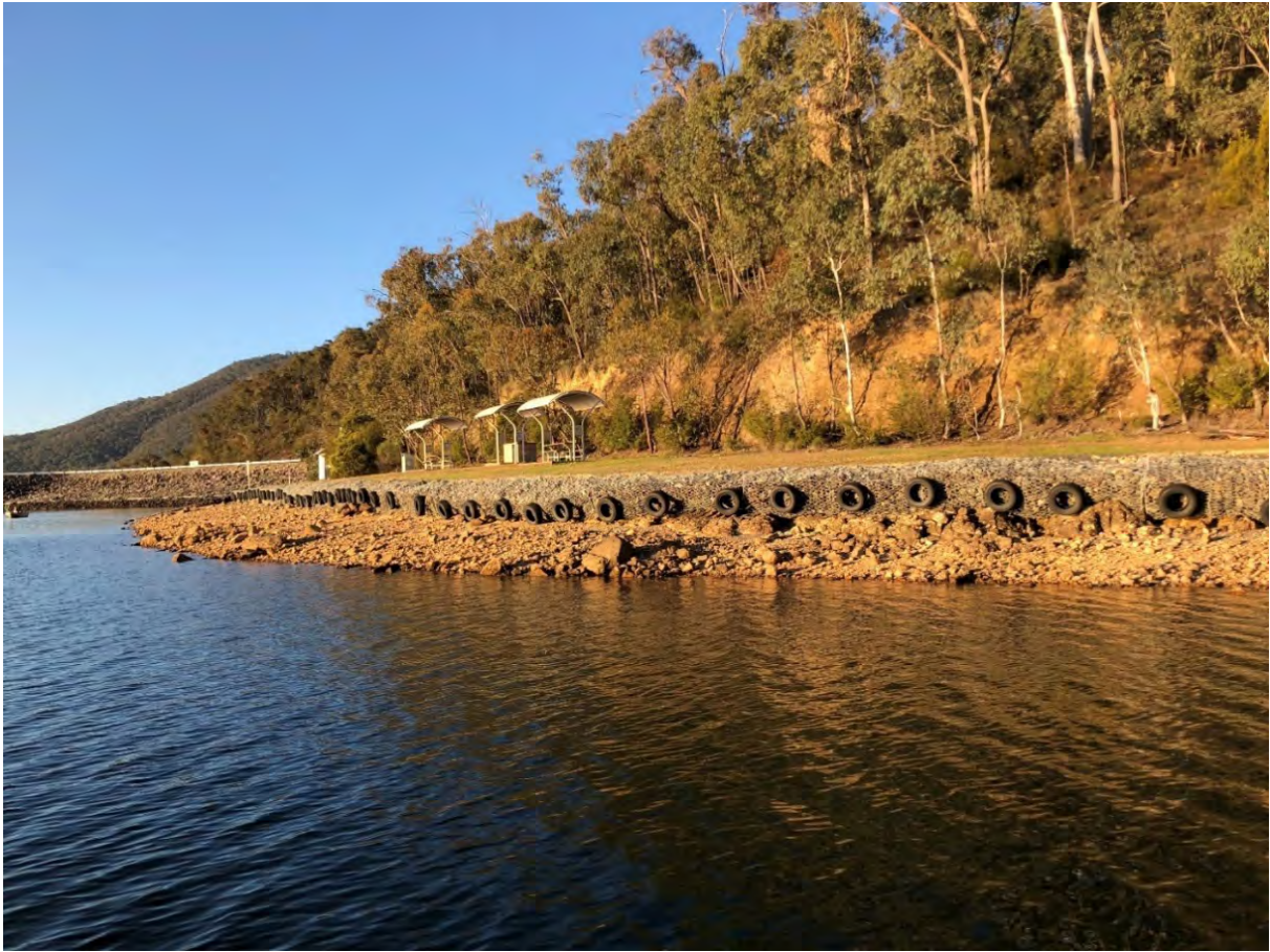
Photograph 3.1 Foreshore area south of the existing boat ramp at Talbingo Reservoir
