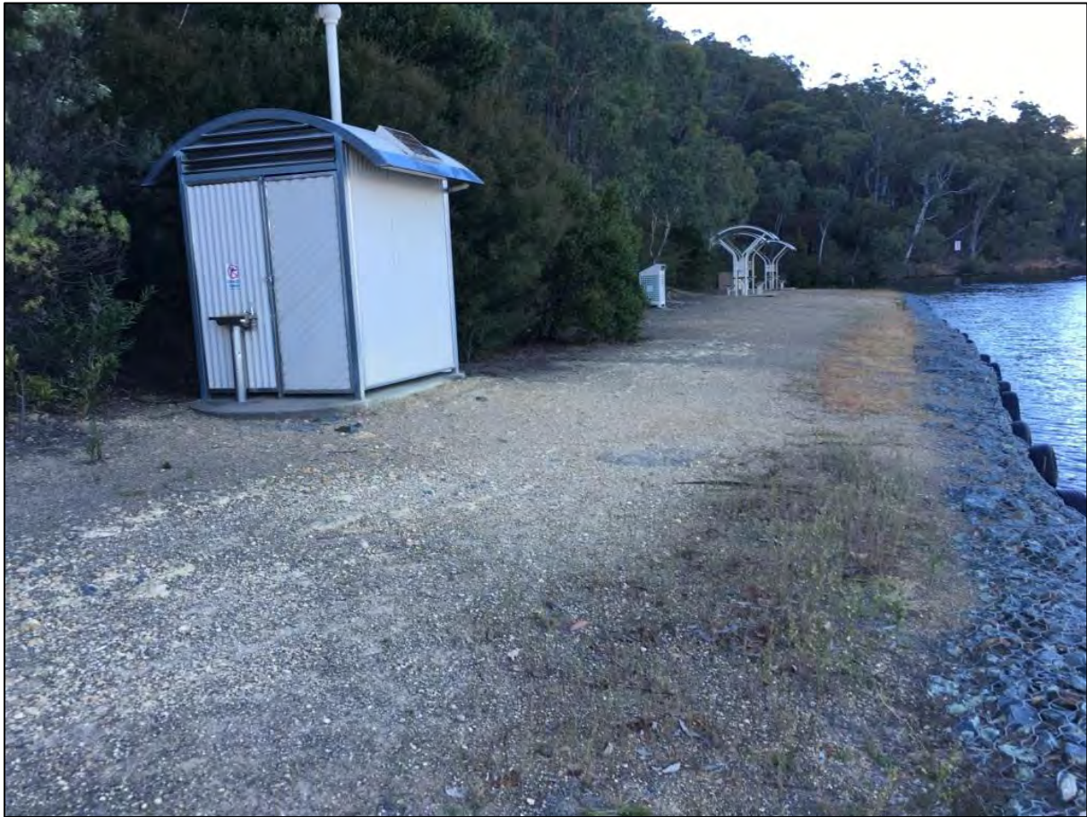
Plate 3.2 Talbingo boat ramp public recreation area
