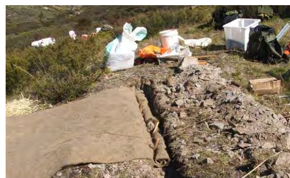
Figure 6-5 Anchoring of jute mesh to stabilise organic matter on a slope
