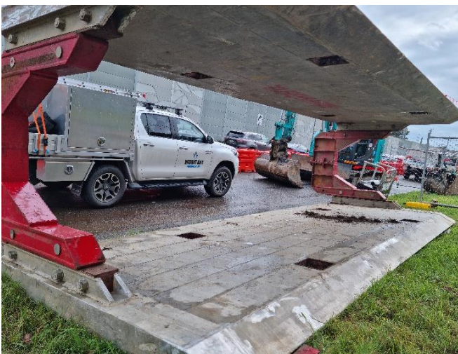
Three large shoring boxes, like the one pictured, will be inserted into the ground between Junction Street and Bridge Street while we install the new stormwater drain. Due to the trench being a deep excavation, these shoring boxes are required to support the sides. As we move up the road, these get moved through the trench to where they are needed.
