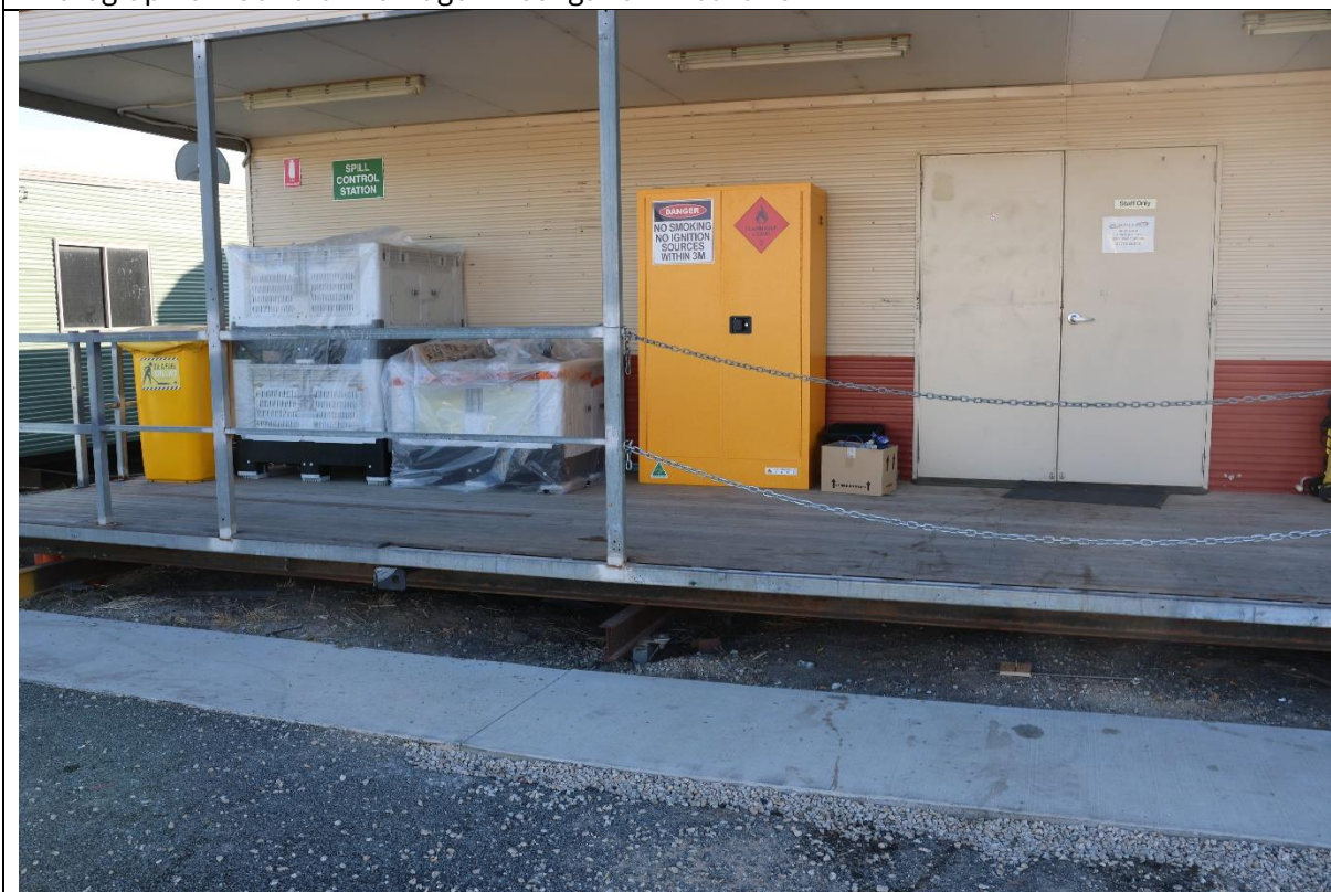
Photograph 6 – Hazardous Materials Storage
