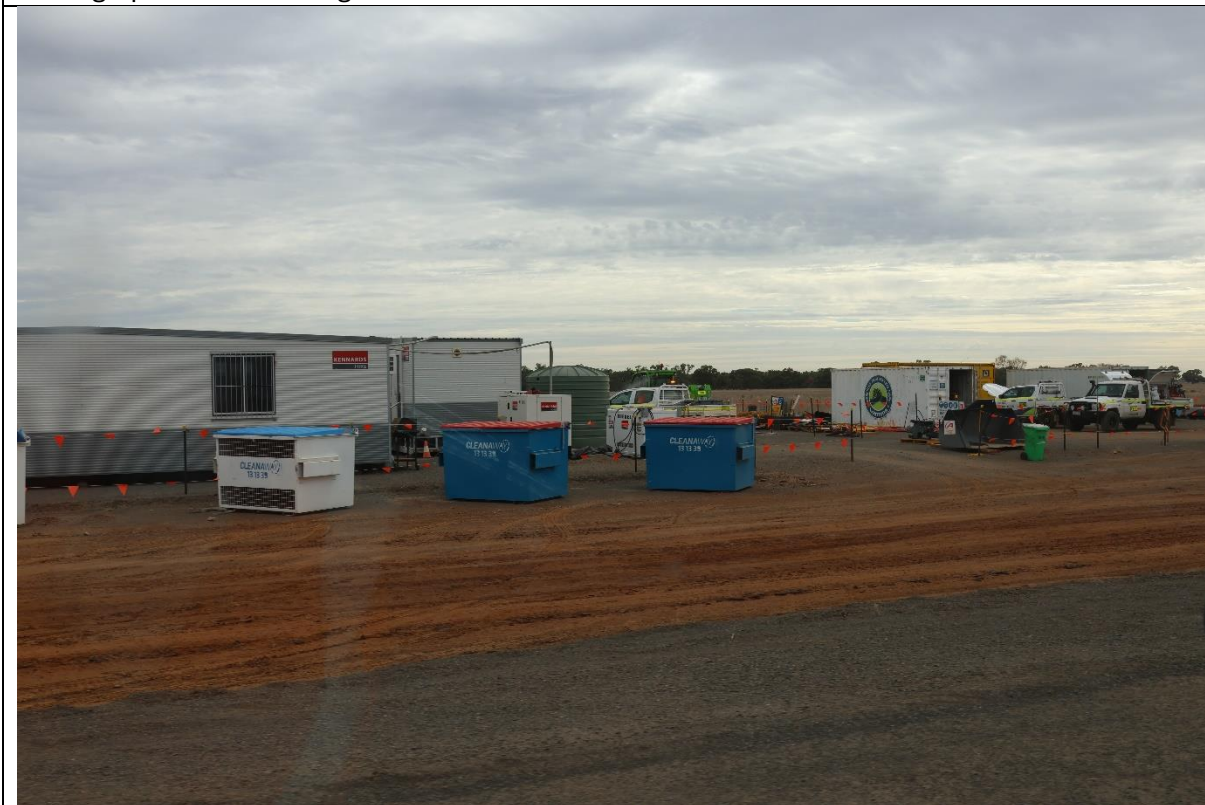
Photograph 8 – Typical Waste Storage
