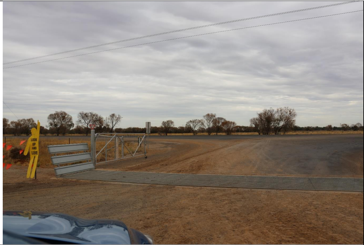
Photograph 1 – Sediment Tracking onto Kidman Way
