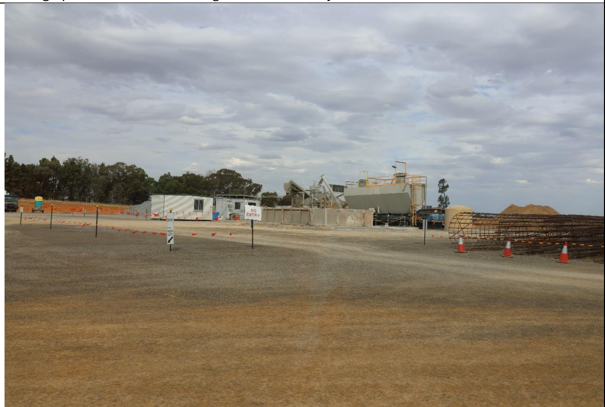
Photograph 2 – On-site concrete batching plant
