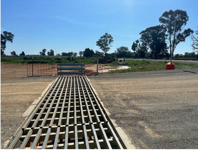
Photo 13: Rumble grid and stabilised access – Camp 2
