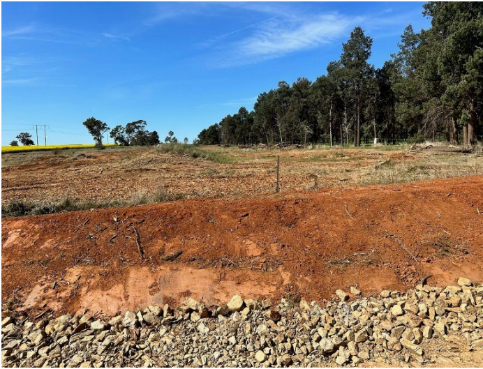
Photo 1: General mainline clearing area
