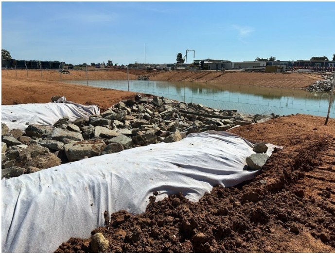
Photo 9: Sediment basin and overflow point
