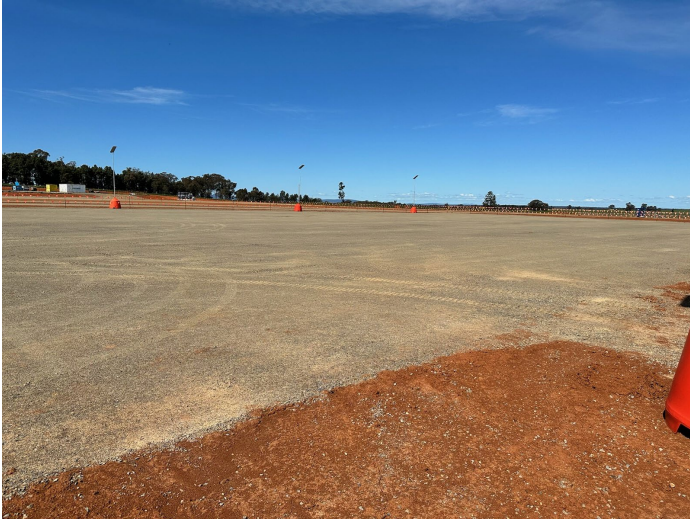
Photo 5: Camp 2 - Laydown area
