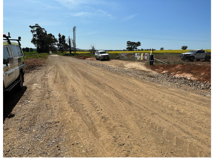
Photo 6: Typical access point and minor road upgrade works
