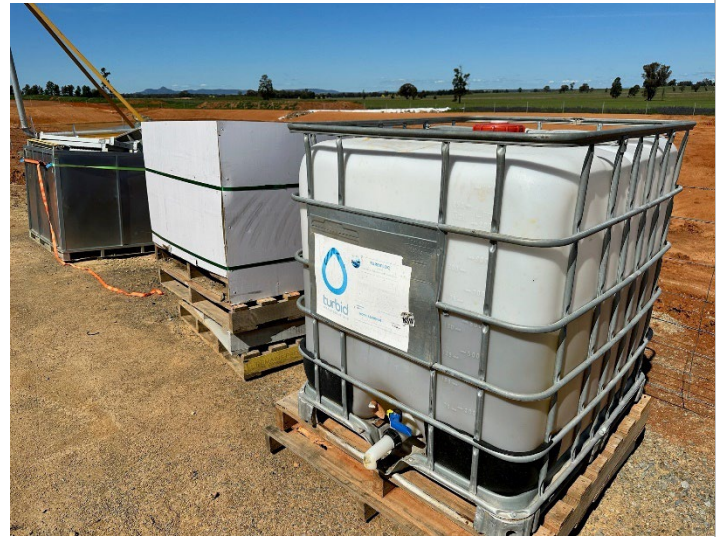
Photo 10: Chemical flocculants for sediment basin
