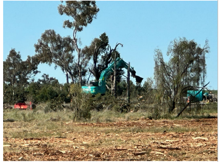
Photo 2: Transmission easement clearing in progress
