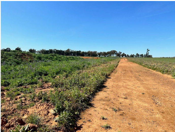
Photo 11: Drainage swale and revegetation (providing groundcover) – Camp 2
