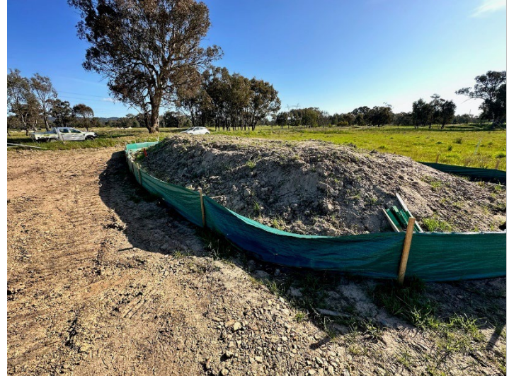
Photo 14: Stockpile < 2m with sediment fence installed
