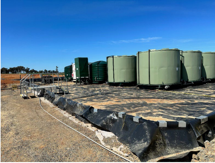
Photo 17: Water treatment plant – Camp 2
