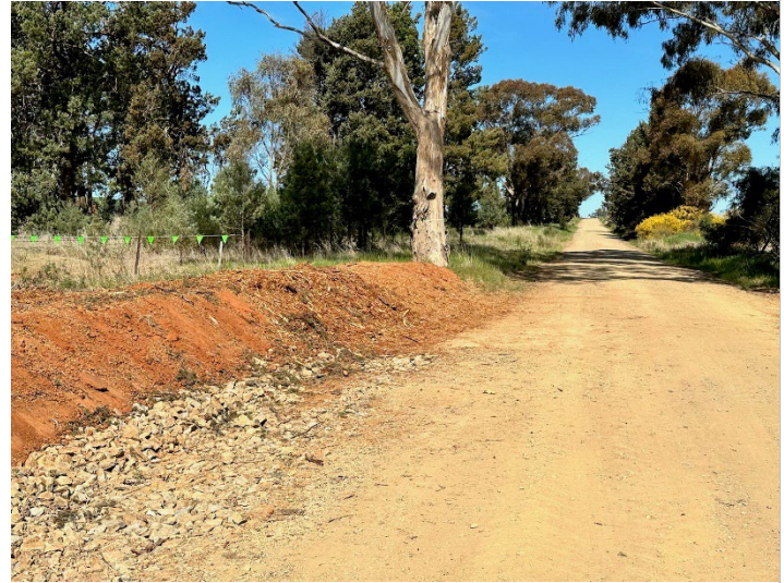
Photo 8: Road adjustment, typical access point
