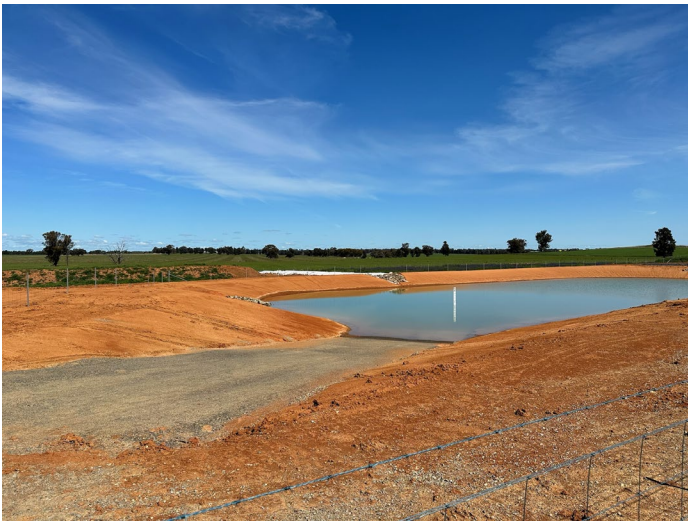
Photo 15: Sediment dam, Camp 2
