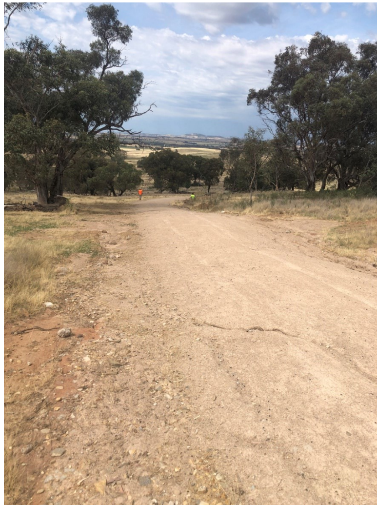
Figure 5-76 Holding H197 track dirt road looking west
