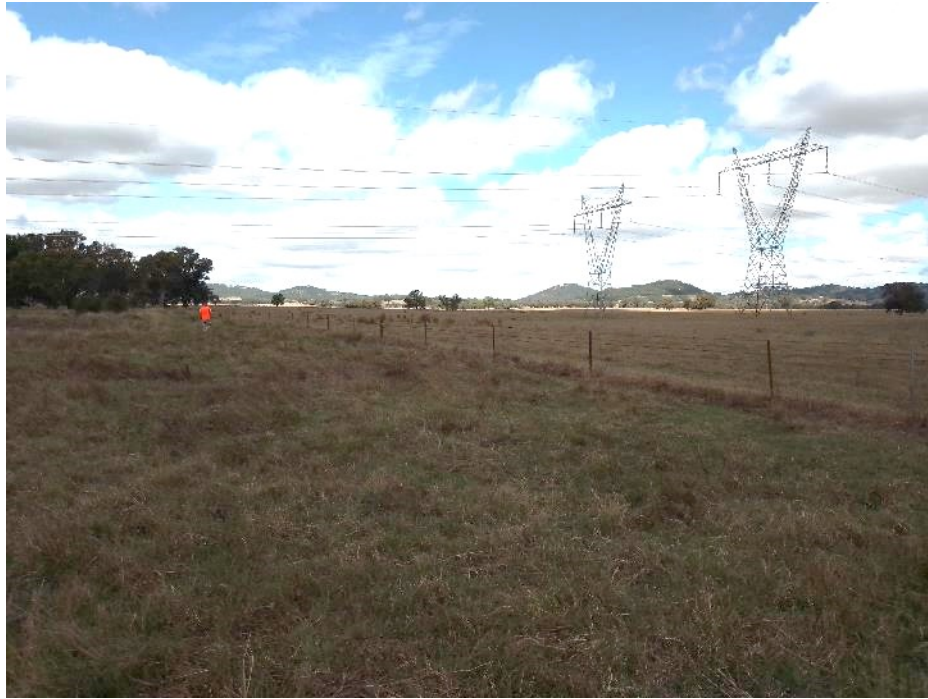
Figure 5-69 Powerline easement at Holdings H208 and H209
