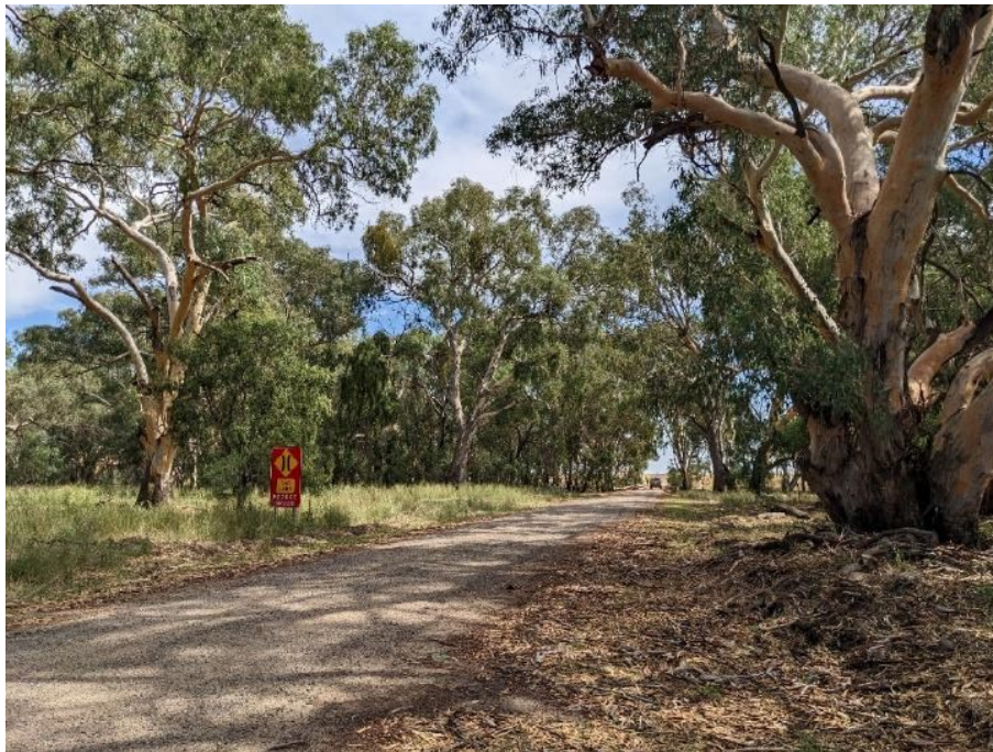
Figure 5-42 Section of the road surveyed near Yanco Creek (view northwest)
