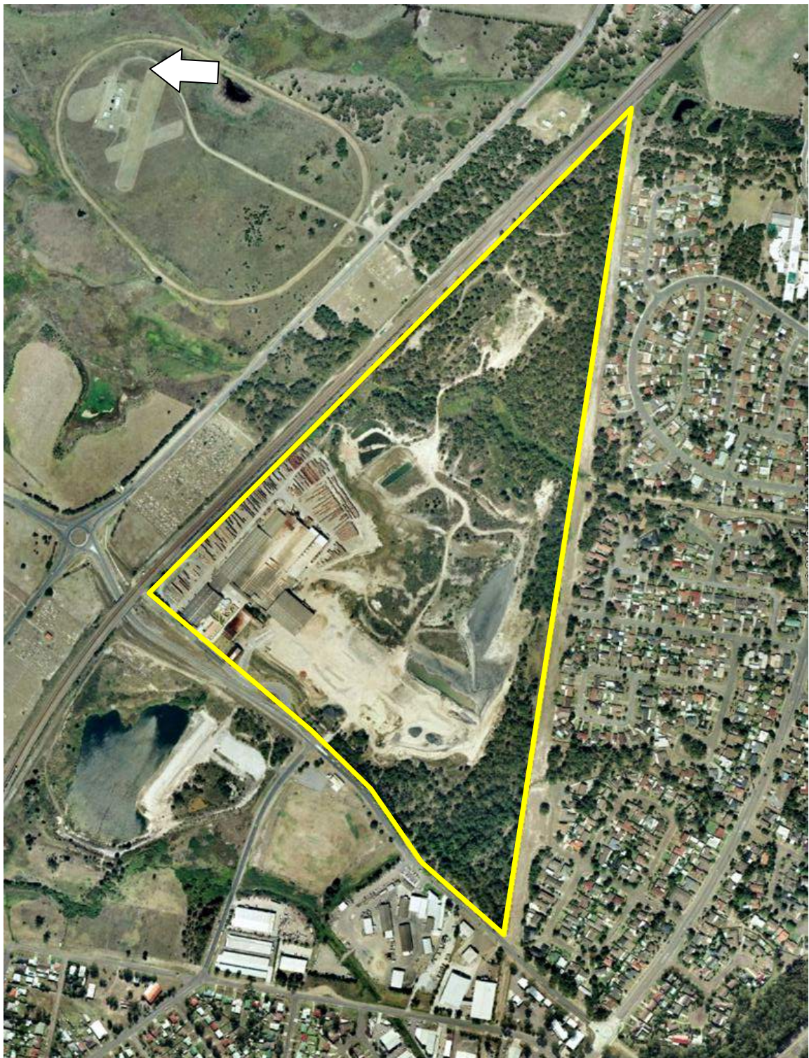
Figure 2 Aerial photograph showing study site (yellow outline).
