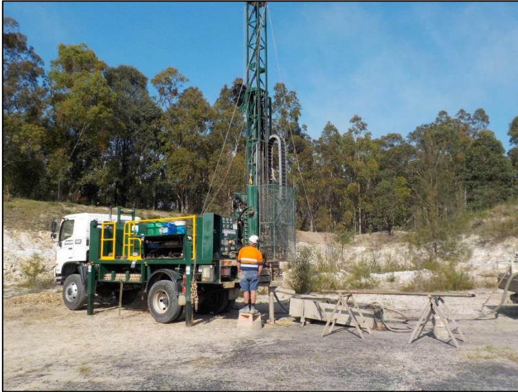
Figure 19: Drilling Rig set up at Borehole 601 (looking west)
