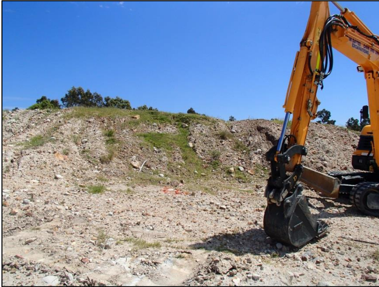
Figure 7: Stockpile adjacent Pit 301, comprising cohesive soils and ripped bedrock (2015)
