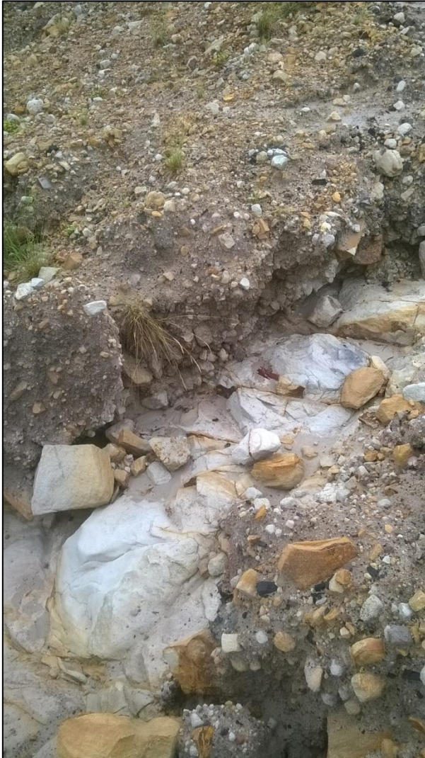
Figure 32: Localised filling underlain by sandstone in quarry batter
