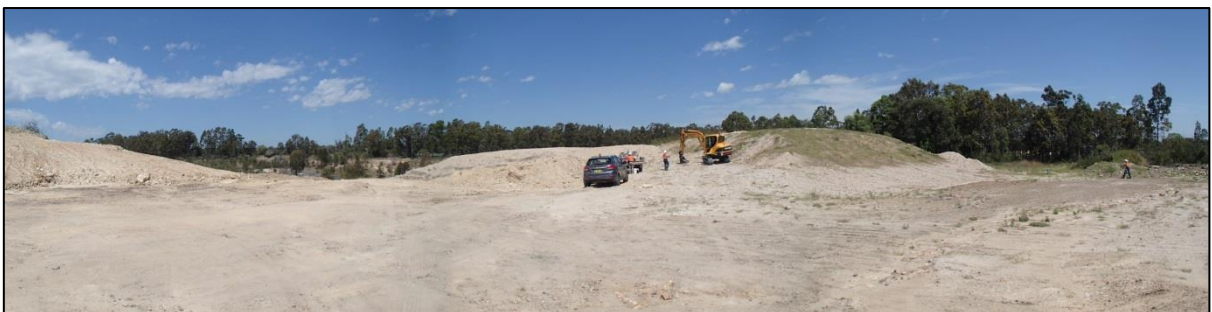
Figure 6: Looking south from the site boundary, excavator at Pit 301 (2015)
