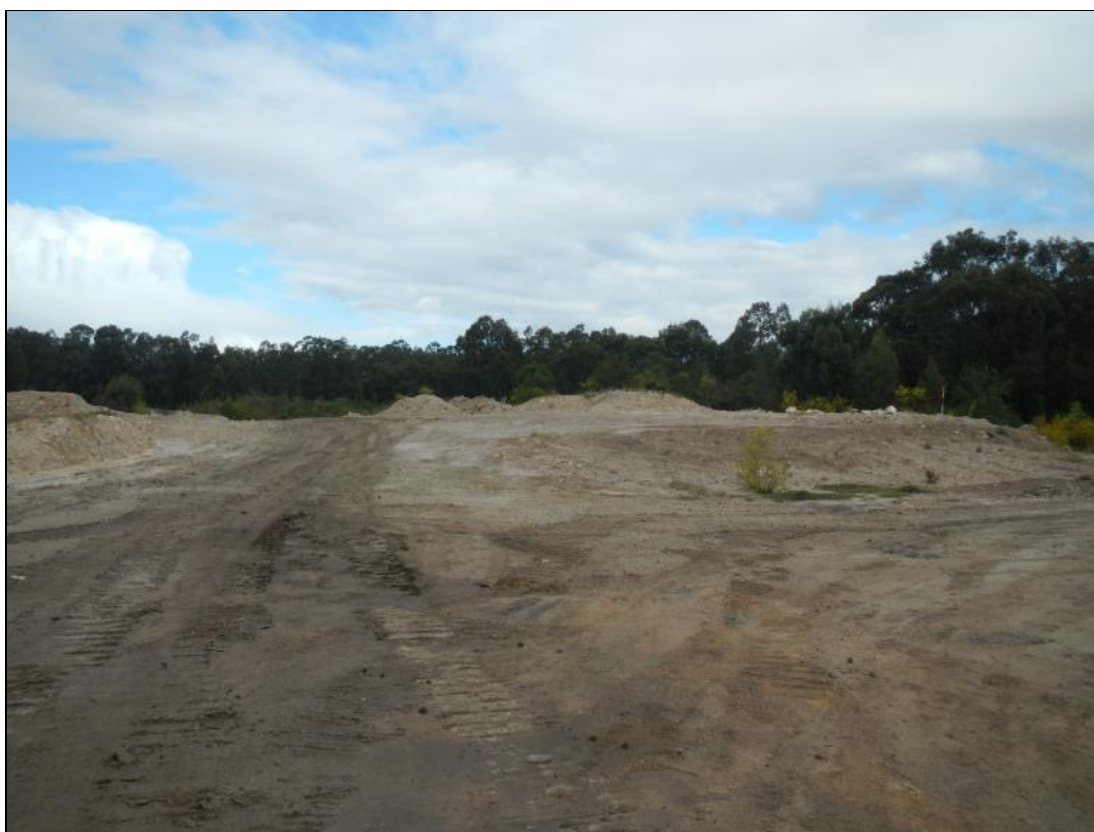
Plate 5.1 View south overlooking portion of project area stripped of topsoil
