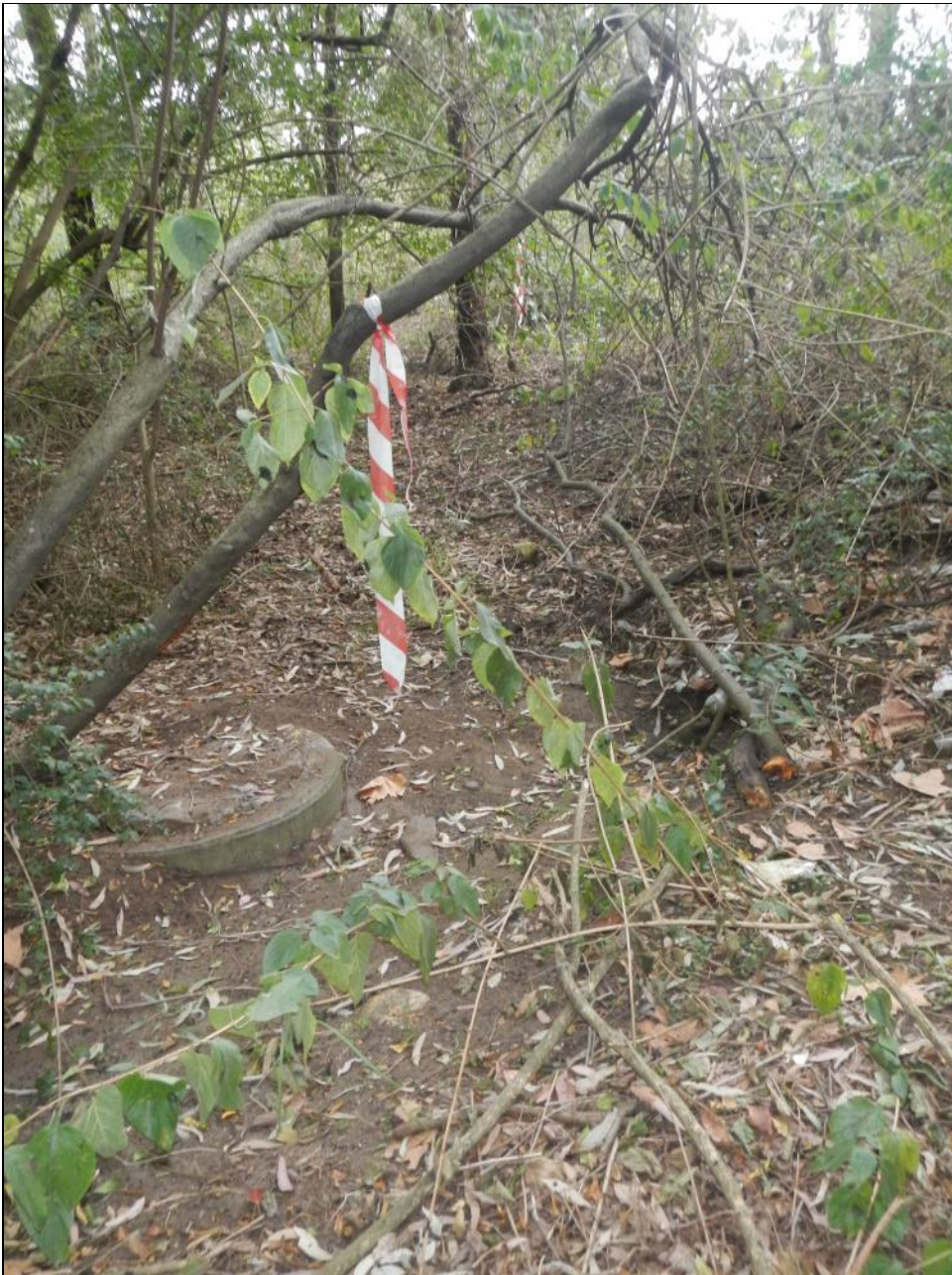
Plate 5.7 View of sub-surface utility and associated cuts
