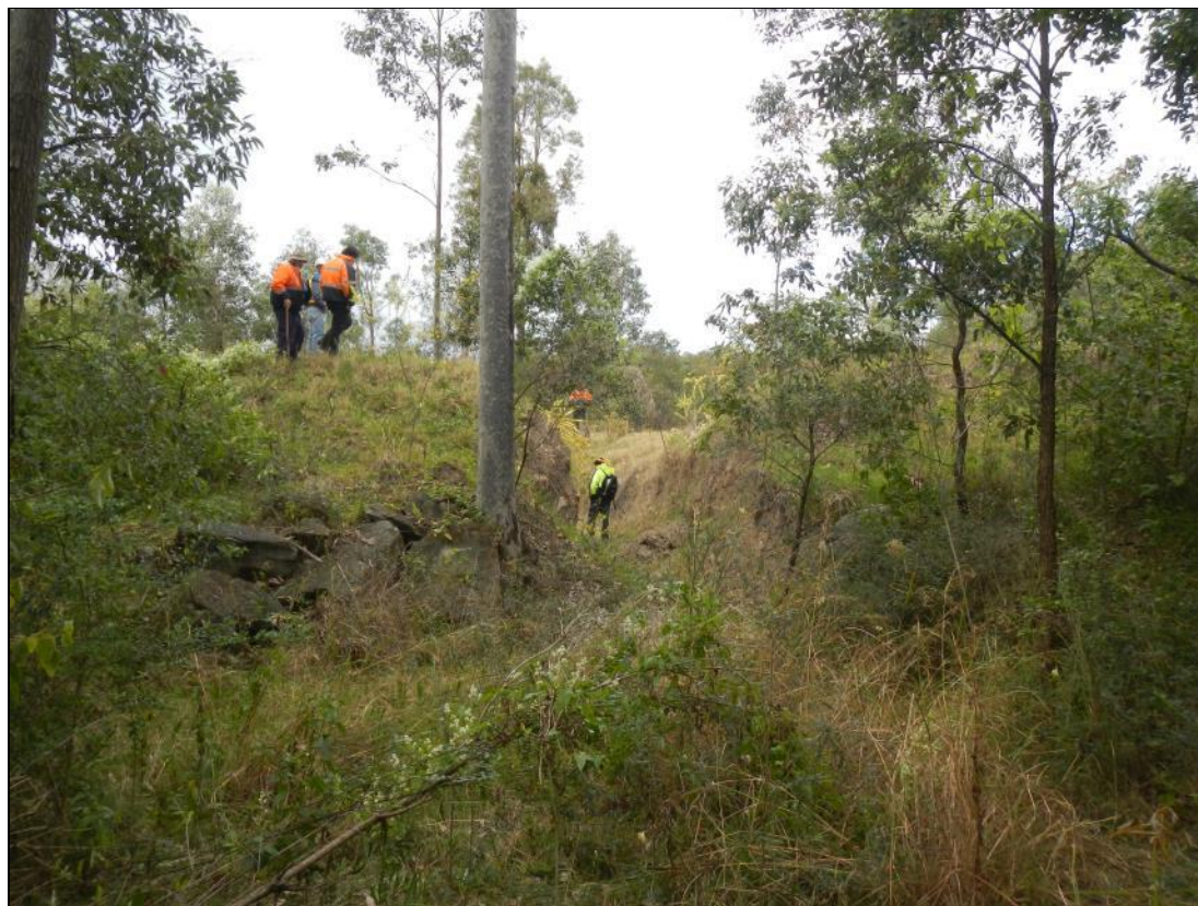
Plate 5.5 Showing cut and soil and boulder dumps
