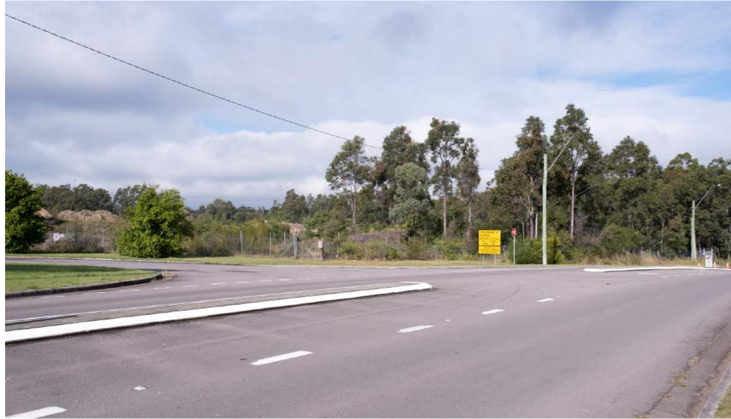
MAIN ENTRY - View from Metford Road looking south-east
