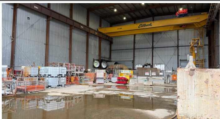
Photo 24: Site compound C1 – C1 Shaft access located within a cladded enclosure (except for the south-east facing wall). Utilised for equipment storage.
