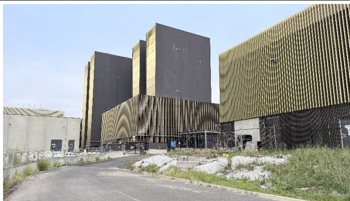
Photo 17: Site Compound C1 – Emission stacks building associated with the ventilation system, constructed in accordance with the M6 Stage 1 Approval
