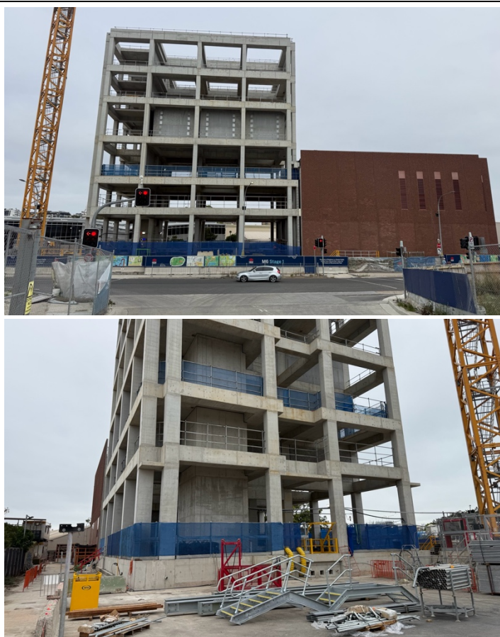
Photo 43-44: Motorway Operational Control (MOC) 3 – Partially constructed MOC 3 building, complete with boundary screening and observed traffic control.
