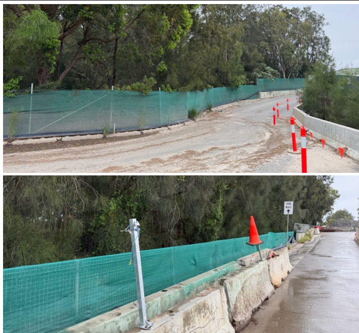
Photo 36-37: Site Compound C3 – Boundary screen adjacent to sensitive area
