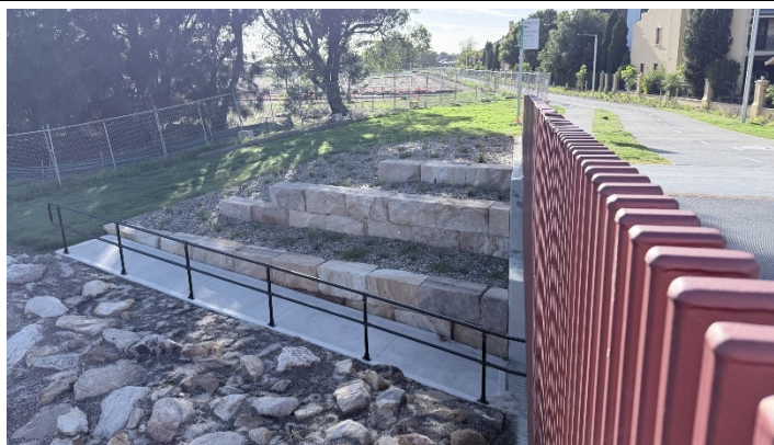
Photo 13: ATL - Bridge over Muddy Creek
