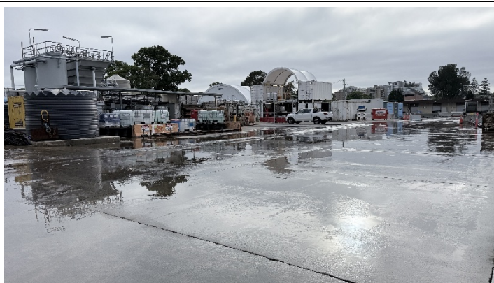
Photo 27: Site compound C2 - Pavements maintained in a clean condition and drainage connected to the site water treatment plant
