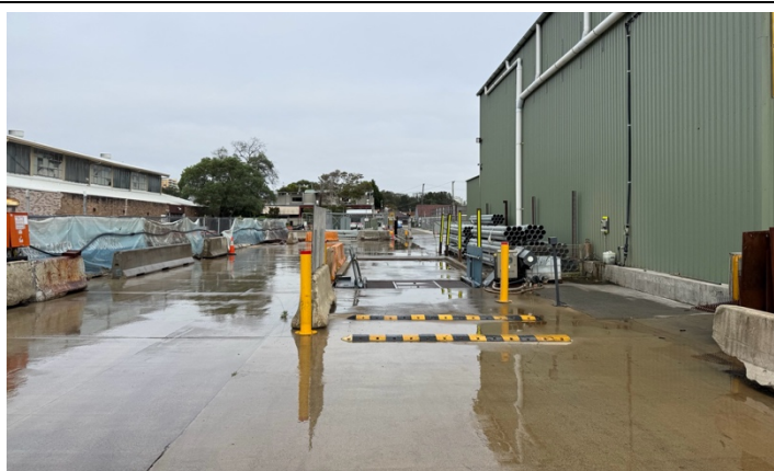
Photo 32: Site Compound C2 – Stabilised site access and wheel wash facility.
