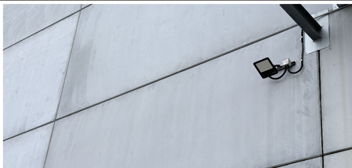
Photo 31: Site Compound C2 - Site Lighting is directed downwards to minimise light spill beyond the boundary of the site compound.
