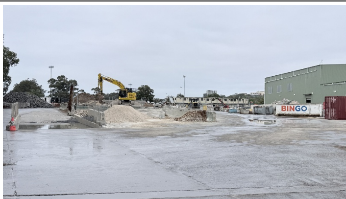
Photo 38: Site Compound C3 – Stockpiled landscaping materials in designated bays.
