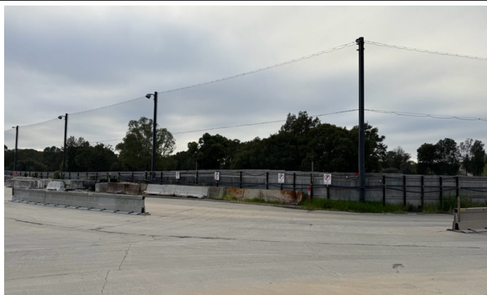
Photo 21: Site compound C1 – Fencing adjacent to the golf course was maintained as a GGBF control.
