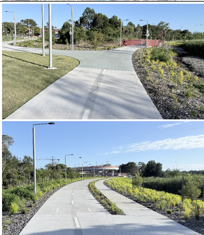
Photos 3 and 4: ATL between Chuter Ave and President Ave.
