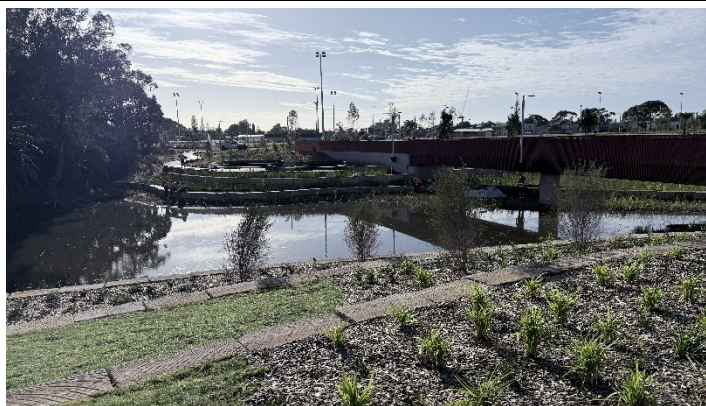
Photos 9 and 10: ATL - Bridge over Bicentennial Park Ponds
