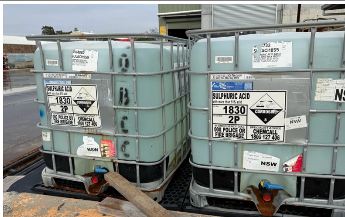
Photo 29: Site compound C2 – Bunded chemical storage adjacent to the water treatment plant.
