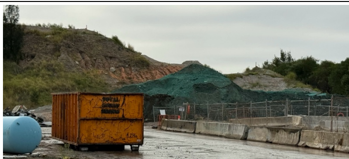
Photo 23: Site Compound C1 - Stockpiled materials treated with polymer prior to the Christmas break.
