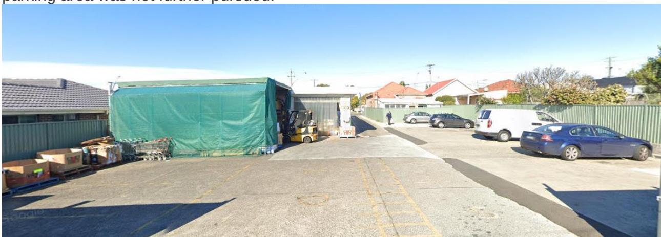
Figure 4: Fruit World onsite parking area from Greens Lane
