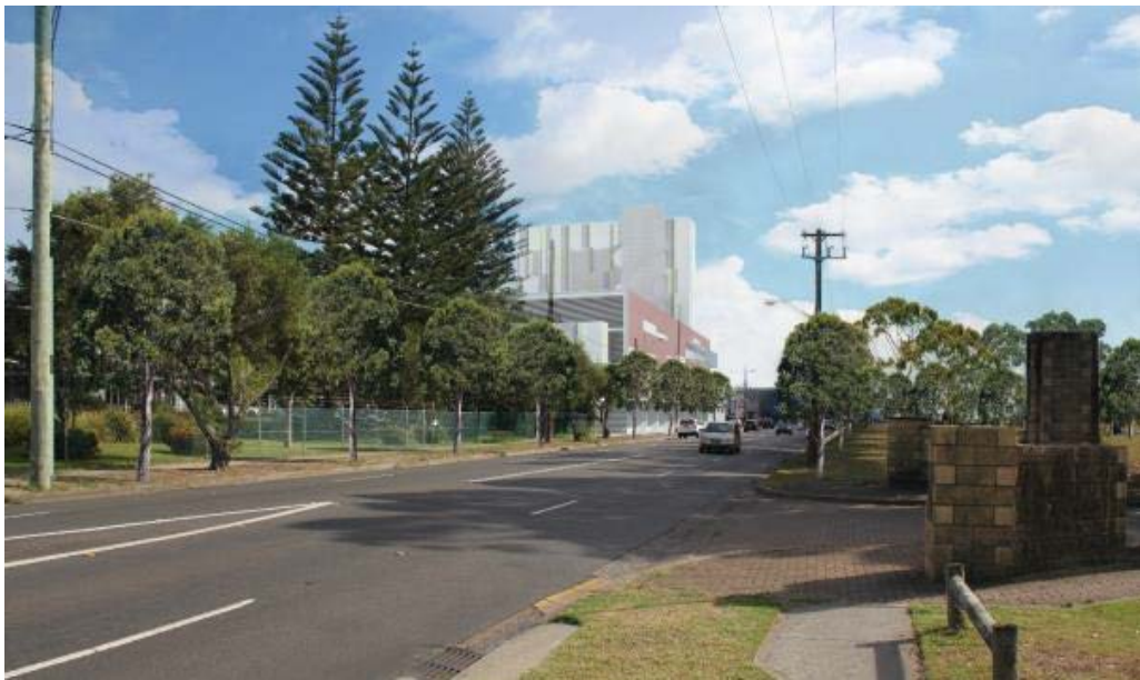
Figure 33 | View north along West Botany Street – Artist's impression during operation (Source: EIS)
