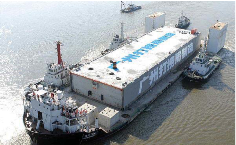
TRANSPORTATION OF AN IMMERSED TUBE TUNNEL ON A SEMI-SUBMERSIBLE VESSEL
