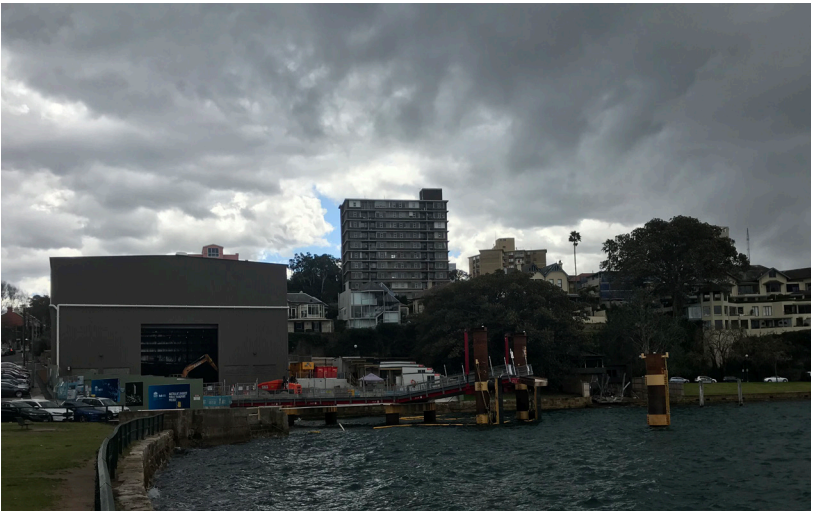
EXAMPLE OF LAND BASED ACOUSTIC SHED AND BARGE ACCESS (SYDNEY METRO BLUES POINT CONSTRUCTION SUPPORT SITE)
