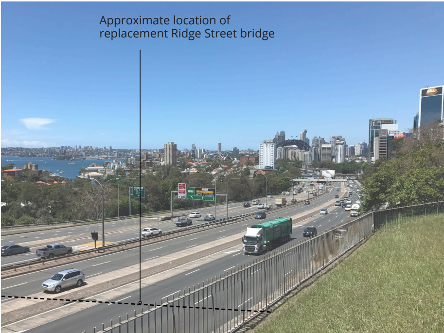
VIEWPOINT 4 - VIEW SOUTH EAST OVER WARRINGAH FREEWAY FROM RIDGE STREET LOOKOUT
