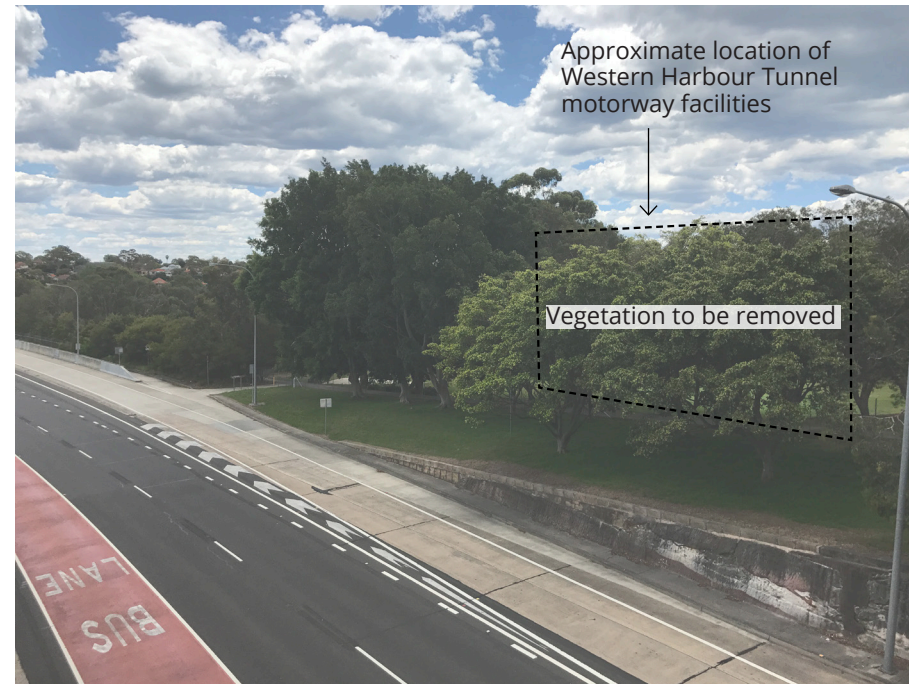
VIEWPOINT 23 - VIEW FROM ERNEST STREET BRIDGE TOWARDS CAMMERAY GOLF COURSE
