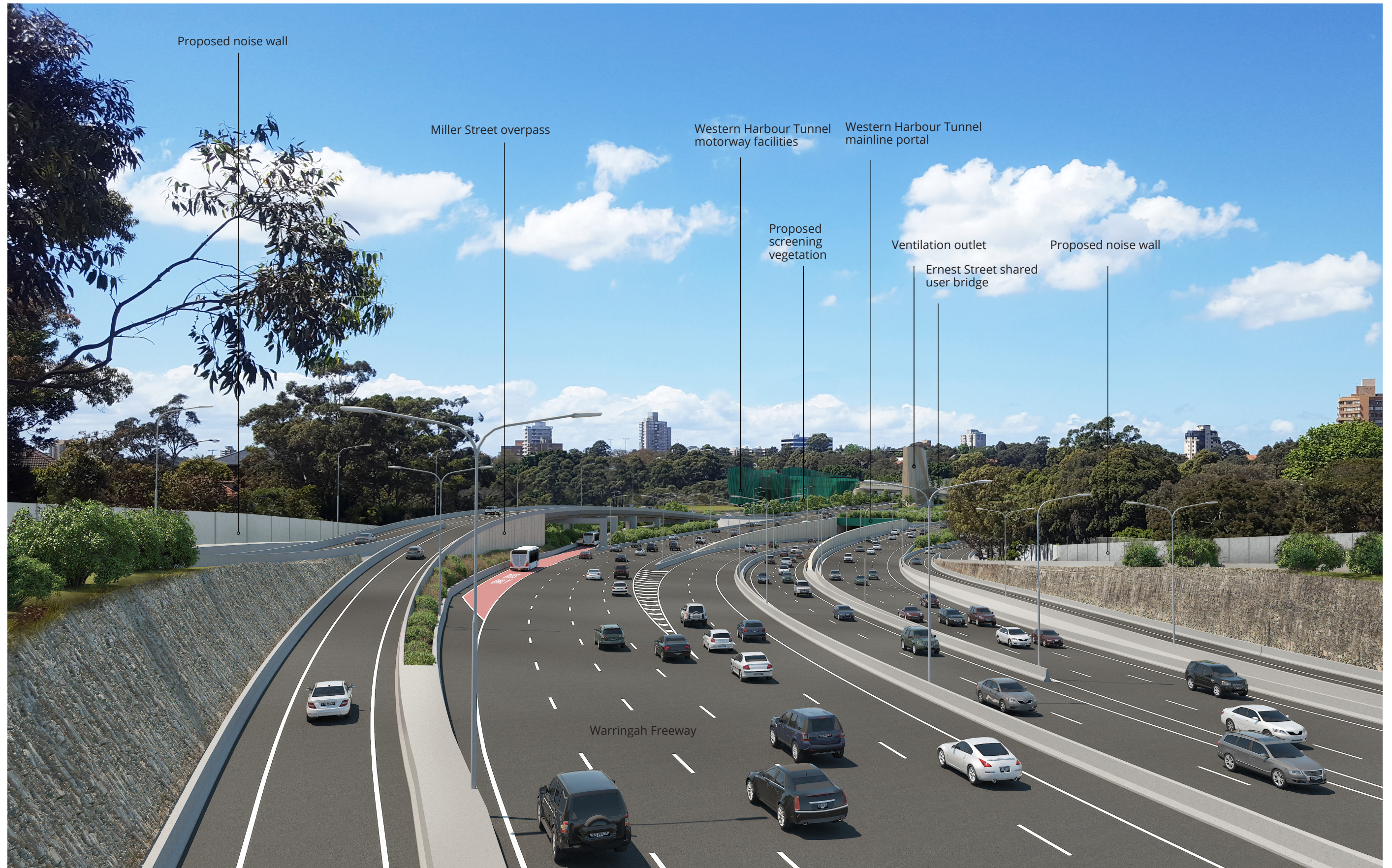
VIEWPOINT 26 - PROPOSED (DAY 1 OF OPERATION) - VIEW SOUTH FROM MILLER STREET BRIDGE
