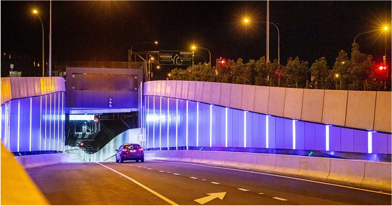
Figure 6-9 Trough structure for New M4 tunnel ramp at Haberfield
