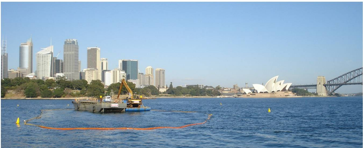
Figure 6-14 Example of backhoe dredger with an open bucket working within Sydney Harbour
