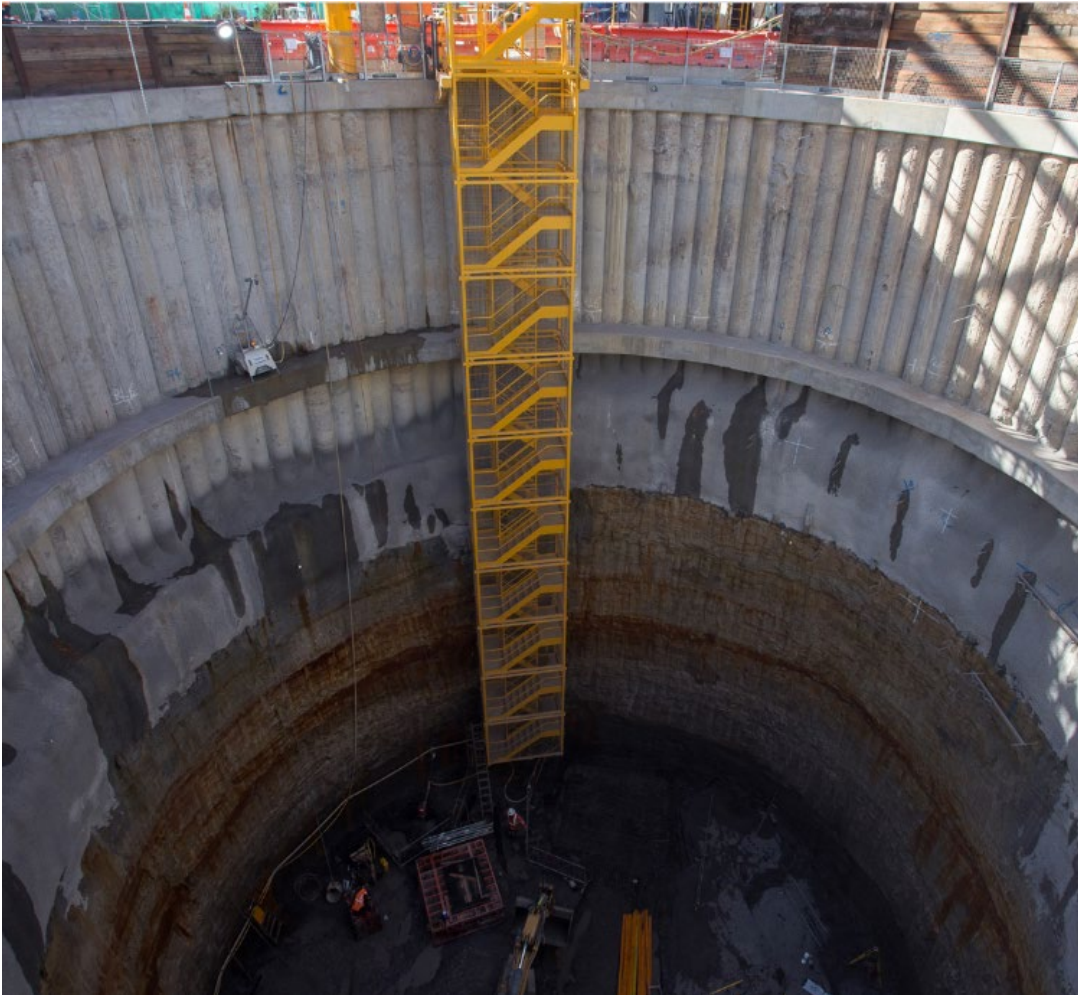
Figure 6-2 Typical tunnel access shaft (Bexley Road New M5, 2017)
