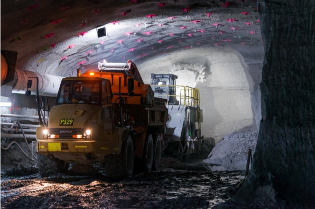
Figure 6-5 Example of a roadheader in the New M4 tunnels loading tunnel spoil into a spoil haulage truck
