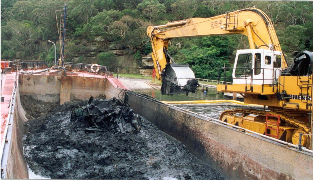
Figure 6-15 Example of an excavator fitted with a closed environmental clamshell loading into a hopper barge
