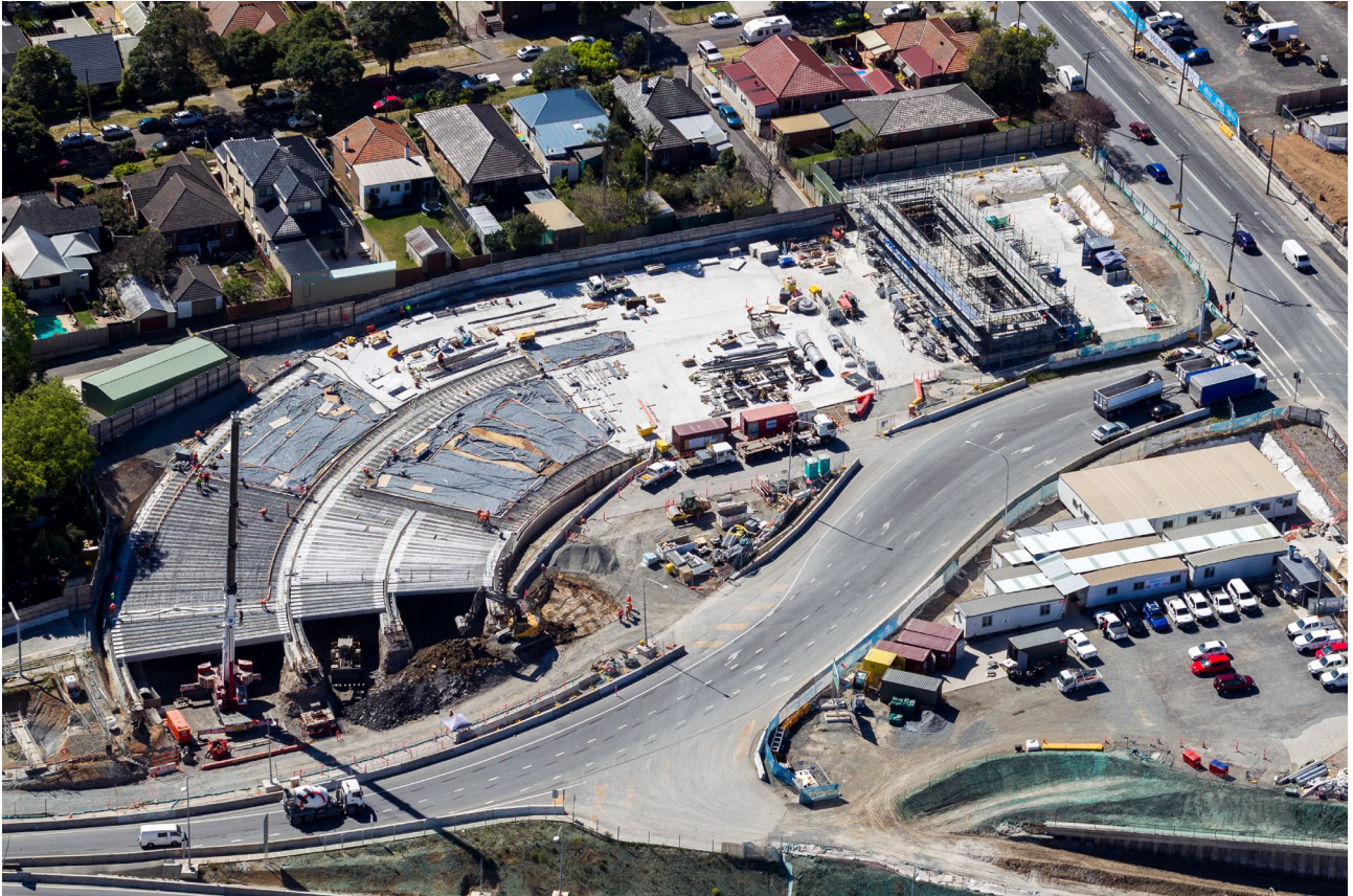
Figure 6-8 New M4 tunnel cut and cover structures
