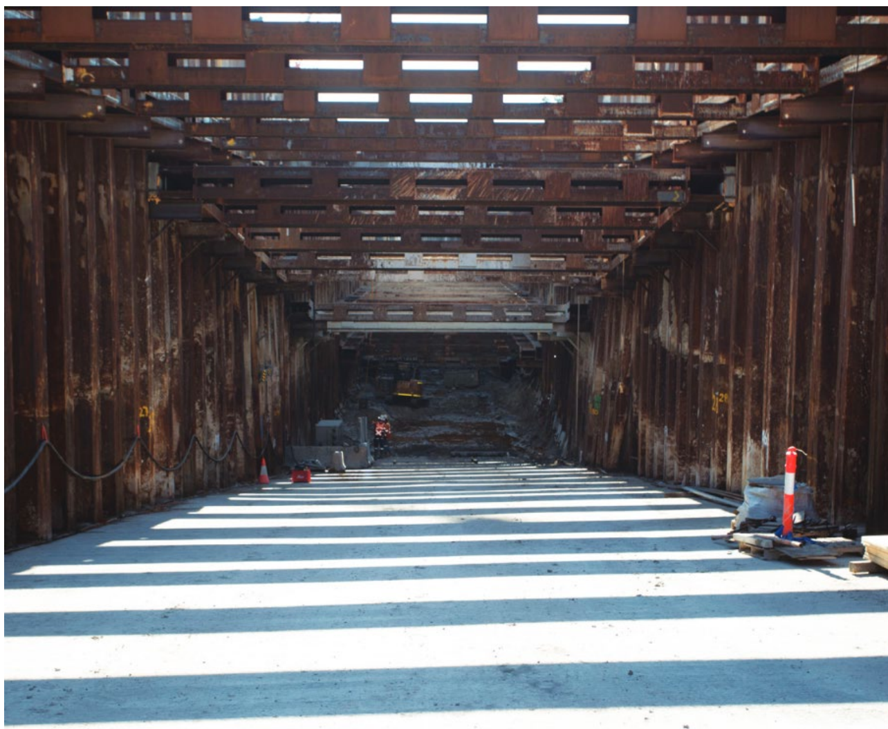
Figure 6-4 Example tunnel access decline (Arncliffe, 2017)
