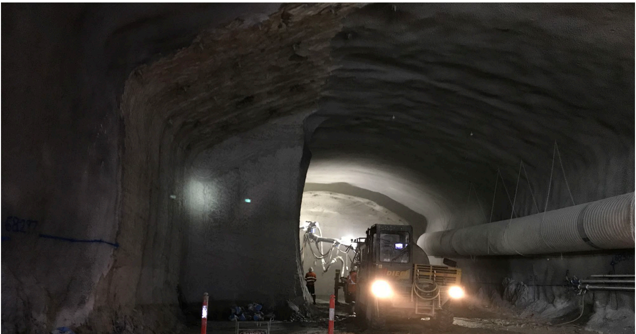
Figure 6-6 Example of tunnel shotcreting
