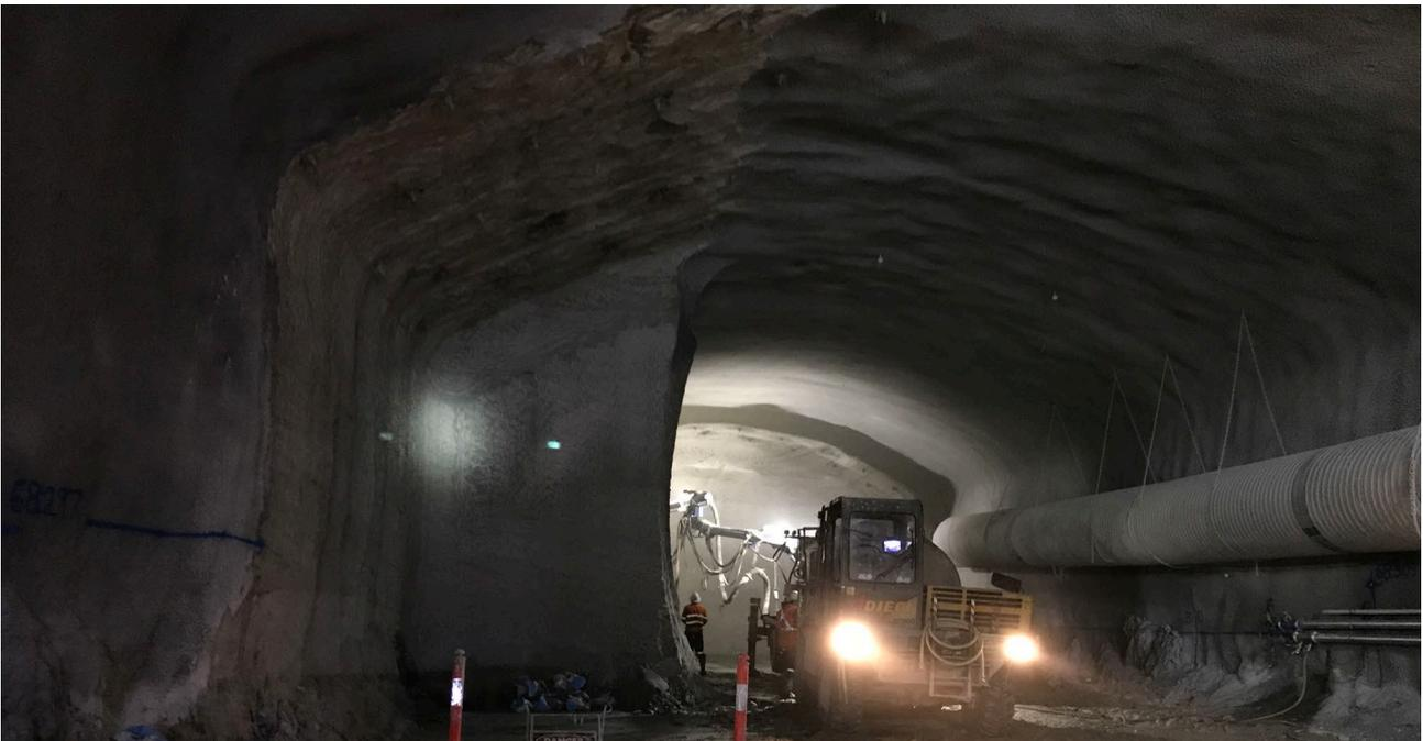
**Figure 6-6** Example of tunnel shotcreting
