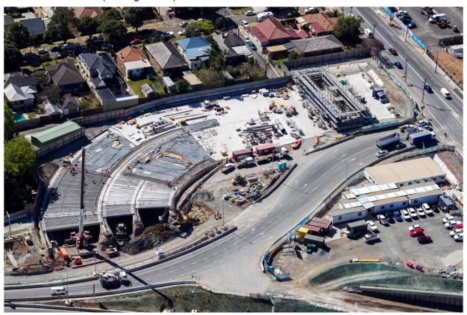
Figure 6-8 New M4 tunnel cut and cover structures
