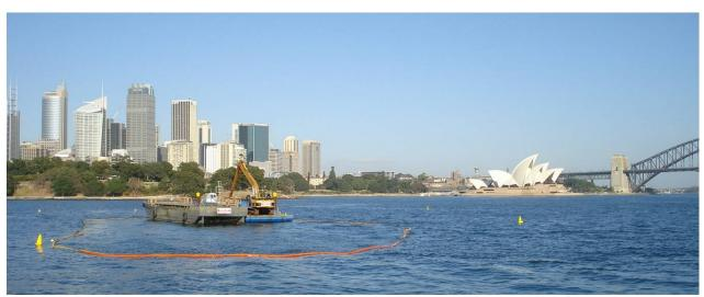
Figure 6-14 Example of backhoe dredger with an open bucket working within Sydney Harbour
