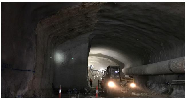
Figure 6-6 Example of tunnel shotcreting
