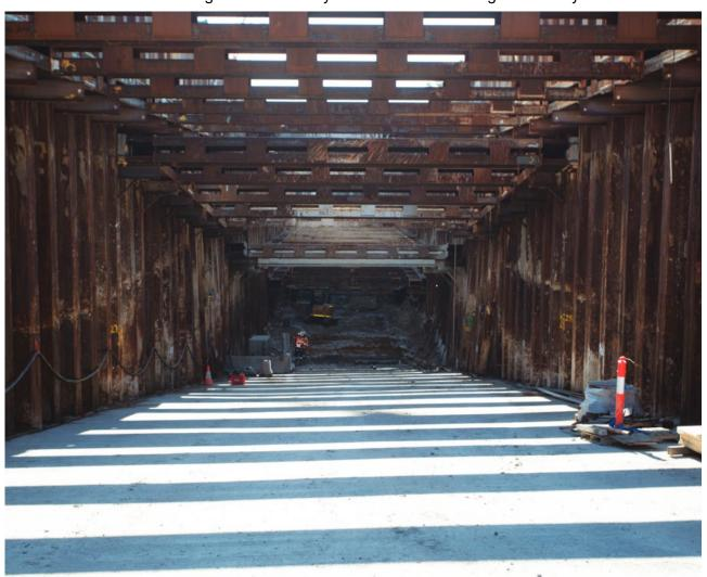
Figure 6-4 Example tunnel access decline (Arncliffe, 2017)
