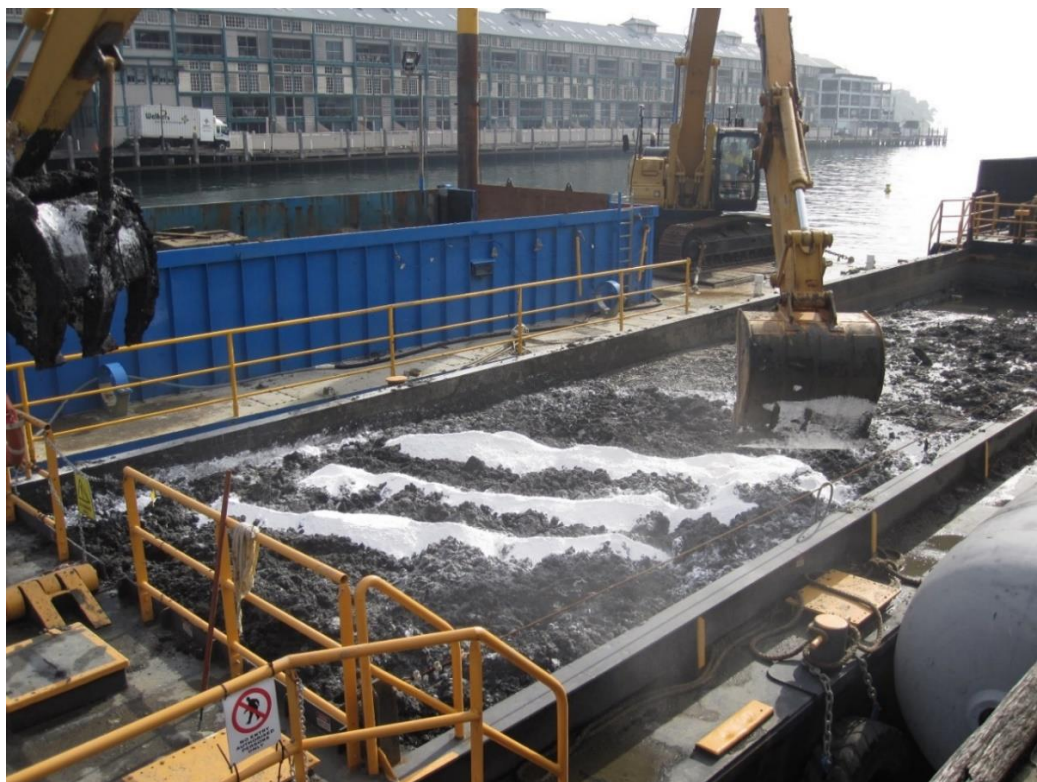
Figure 5-3 Example of material not suitable for offshore disposal being made spadable within a barge at Potts Point for the Garden Island dredge works in 2010 (Source: Royal Haskoning)
