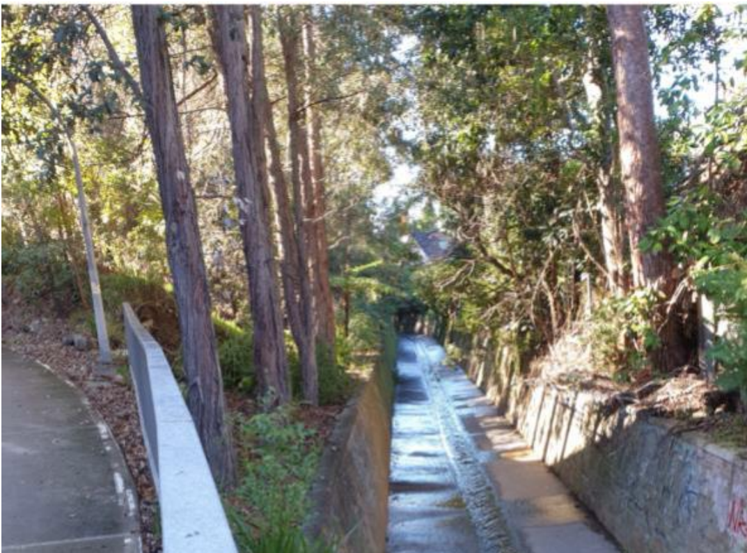
Figure 2-10 Example of a section of Flat Rock Creek classified as lined contributing baseflow near Glenview Road at Naremburn (FRC015)
