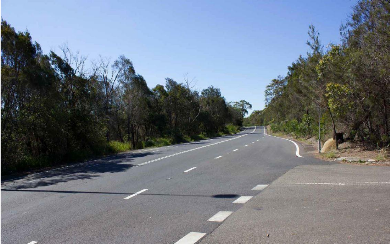
Figure 22-26 Existing view north along Wakehurst Parkway near Kirkwood Street
