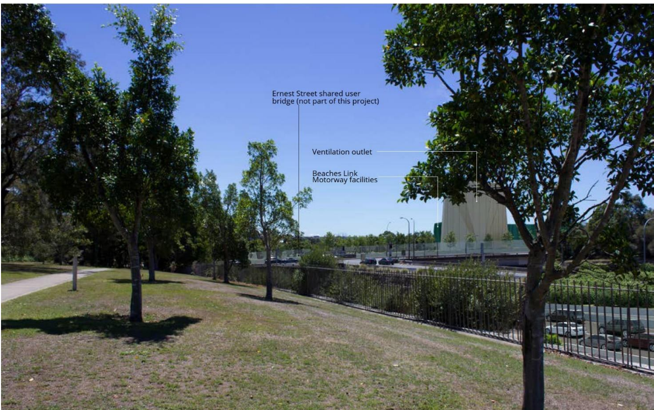
Figure 22-12 Proposed view (year 1 of operation) north east over Warringah Freeway from Jeффreson Jackson Reserve
