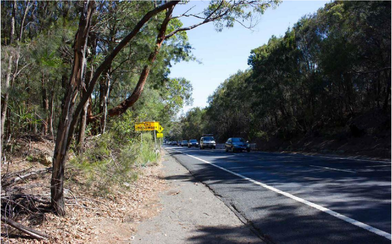
Figure 22-28 Existing view south along Wakehurst Parkway near the Warringah Aquatic Centre
