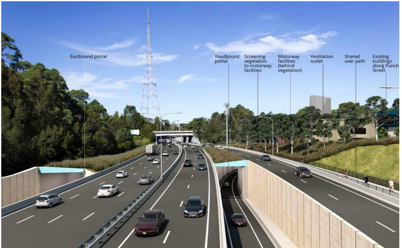
Figure 22-19 Proposed view (year 10 of operation) east over Gore Hill Freeway from Hampden Bridge towards the motorway facilities and ventilation outlet
