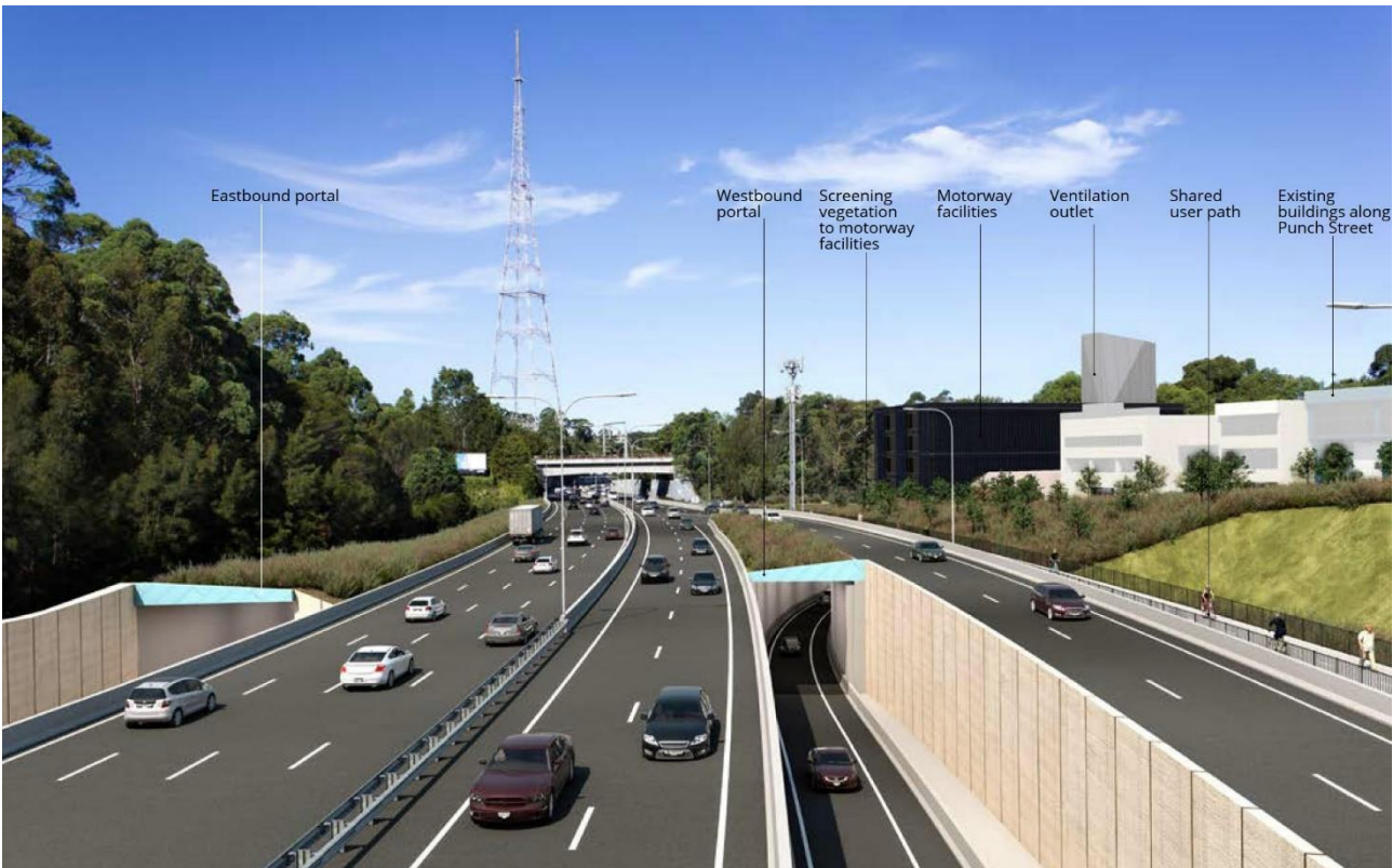
Figure 22-18 Proposed view (year 1 of operation) east over Gore Hill Freeway from Hampden Bridge towards the motorway facilities and ventilation outlet
