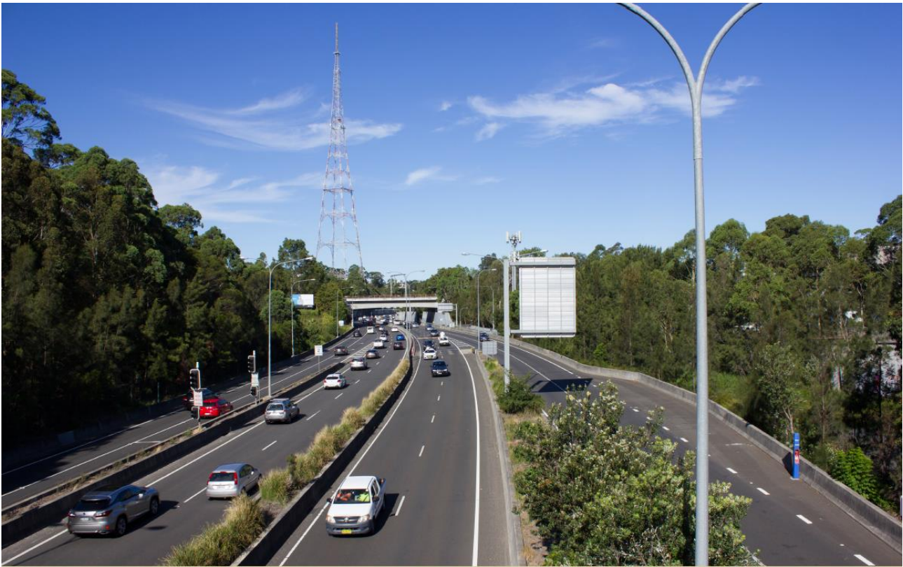
Figure 22-17 Existing view east over Gore Hill Freeway from Hampden Bridge towards the motorway facilities and ventilation outlet
