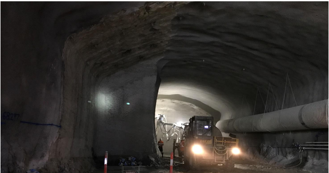
Figure 6-5 Example of tunnel shotcreting
