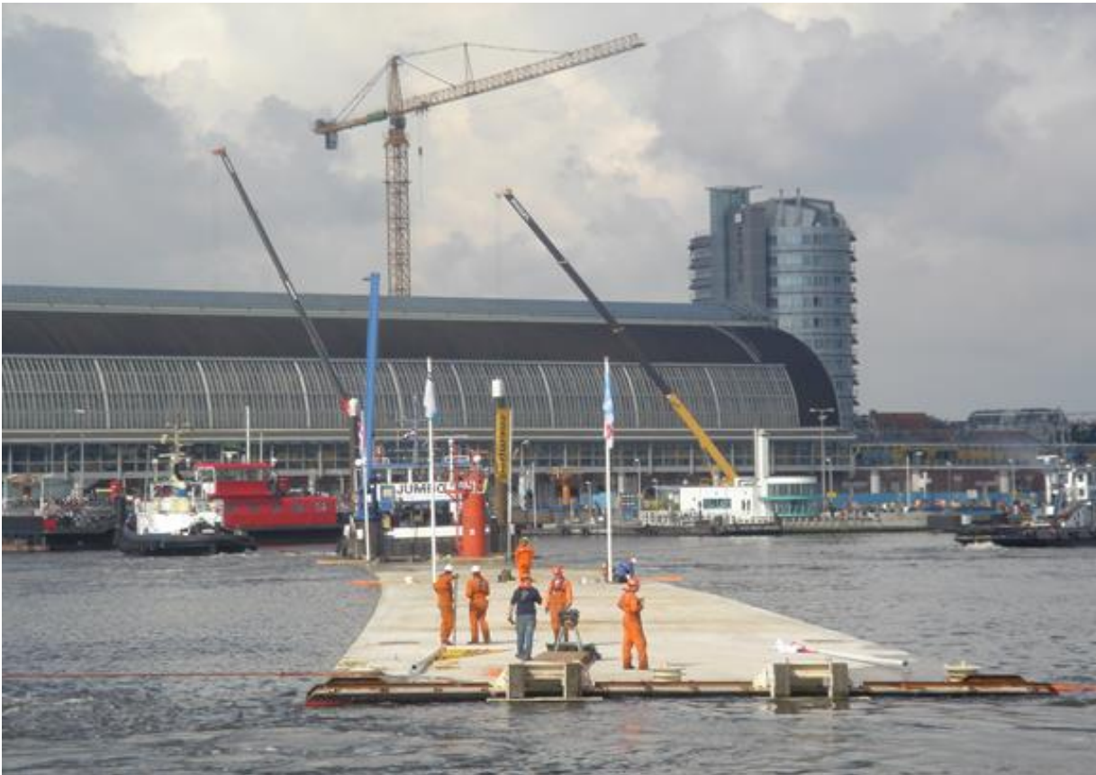
Figure 6-17 Example of completed immersed tube tunnel unit for the Amsterdam Metro moored ahead of installation (Source: ITA, n.d.)
