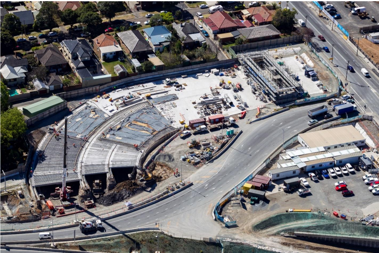
Figure 6-7 New M4 tunnel cut and cover structures
