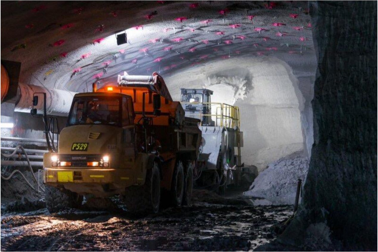
Figure 6-4 Example of a roadheader in the New M4 tunnels loading tunnel spoil into a spoil haulage truck
