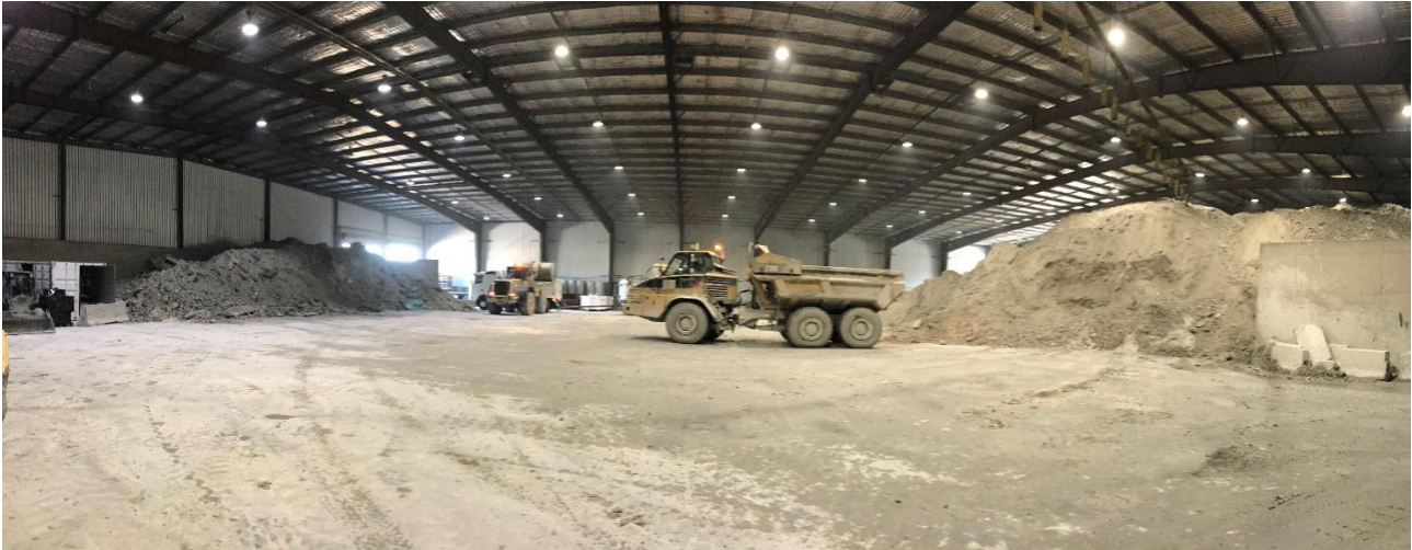
Figure 6-3 Example from within an acoustic shed constructed for the New M4 tunnels
