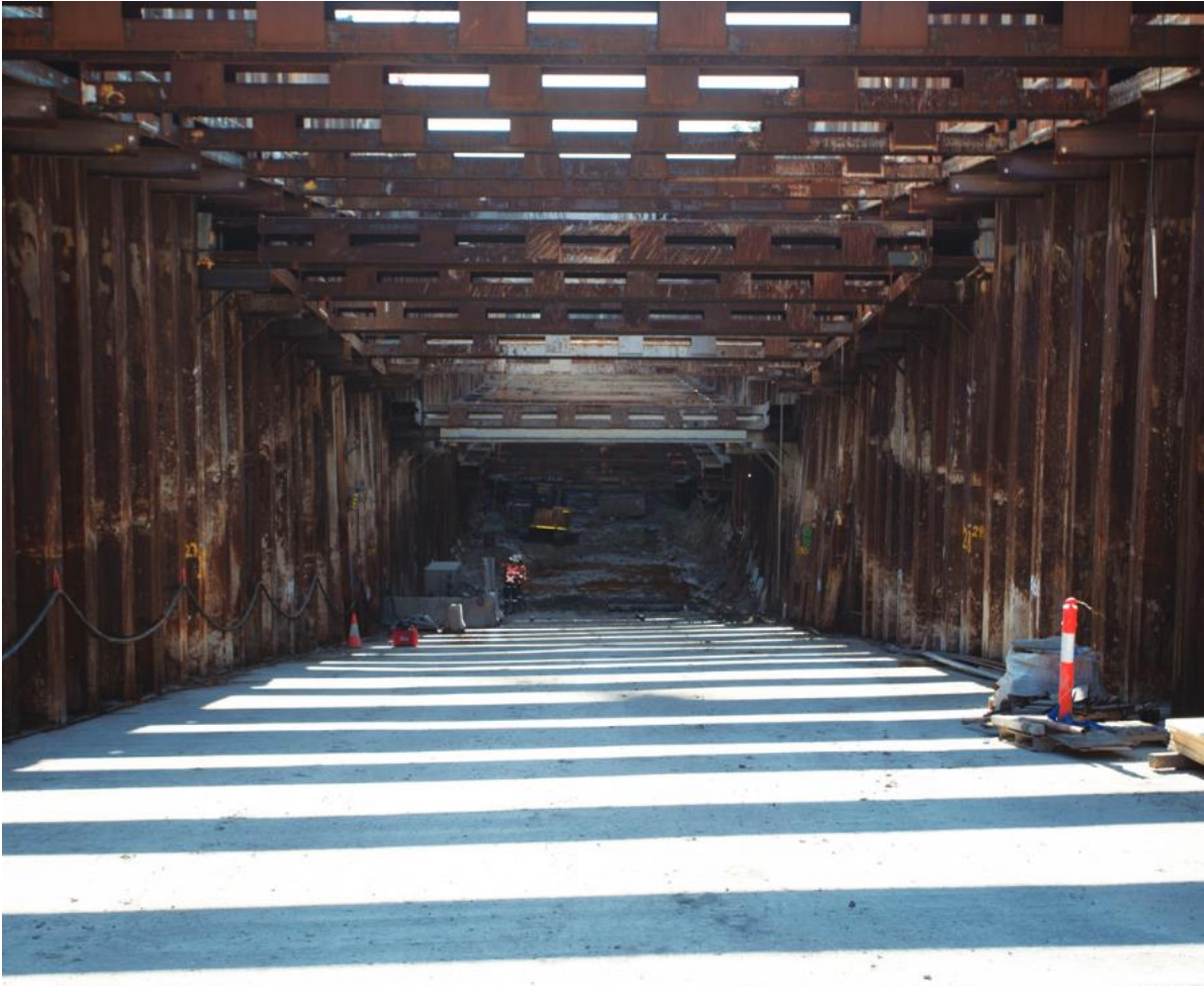
Figure 6-2 Example tunnel access decline
