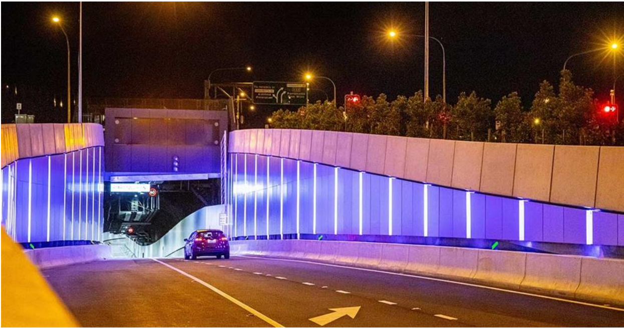
Figure 6-8 Trough structure for New M4 tunnel ramp at Haberfield
