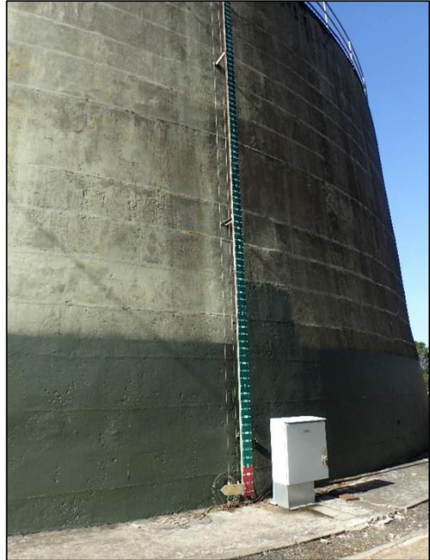
Figure A.12.5 Detail of the water level measure and fuse box attached to the Bantry Bay Reservoir (WS 0008)
