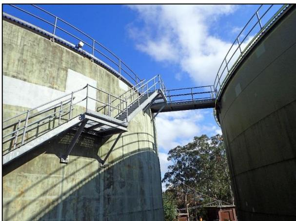
Figure A.12.6 Metal staircase attached to Bantry Bay Reservoir (WS 0008), and catwalk connecting the two reservoirs
