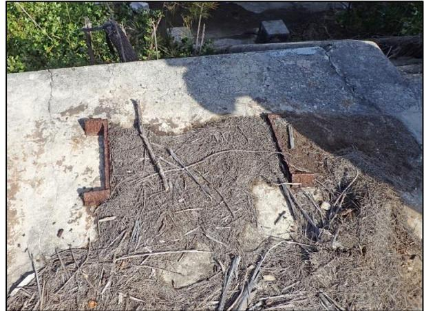
Figure A.12.9 Detail of the rusted metal embedded at the top of the concrete staircase, facing north towards the Bantry Bay Reservoir (WS 0008)
