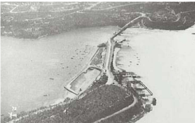
Figure 5-11: Spit Bridge, 1932, showing reclamation (John Hall & Co. 1932)
