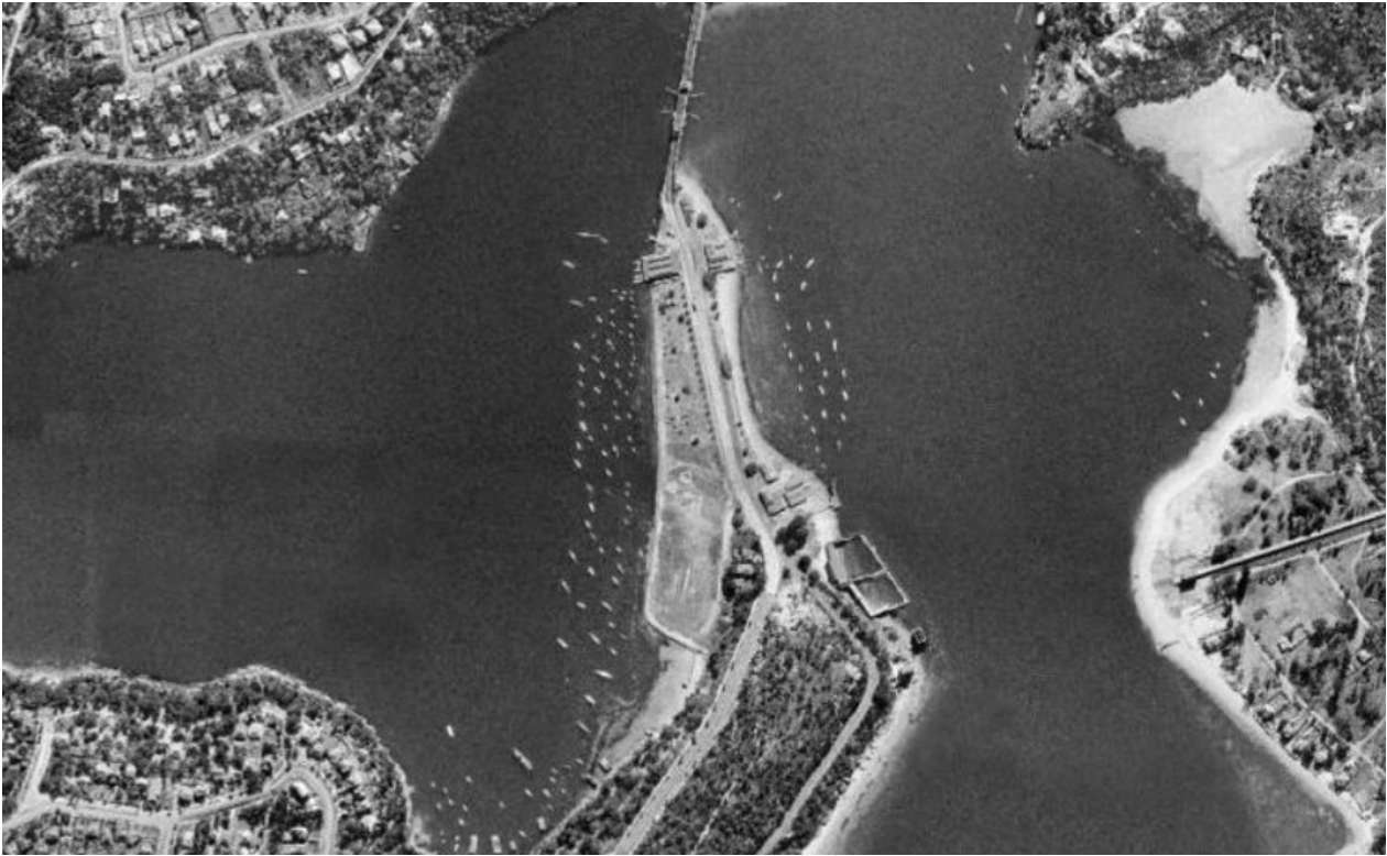
Figure 5-12: 1943 aerial photograph showing the reclaimed land and seawall on the western side of The Spit (RTA Photography 1943). Note the number of moored vessels in Pearl Bay
