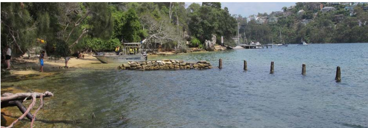
Figure 4-21: West end of Clive Park Tidal Pool showing coarsely stacked sandstone blocks (Cosmos Archaeology 18 December 2017)
