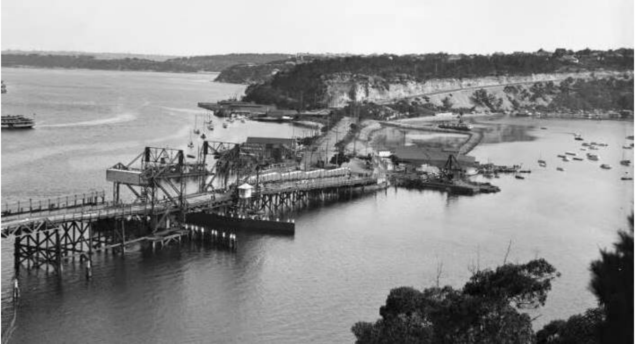
Figure 5-9: ca. early 1930s photograph of Spit Bridge showing reclamation works being carried out on the western side of The Spit (Foster ca. 1930s)
