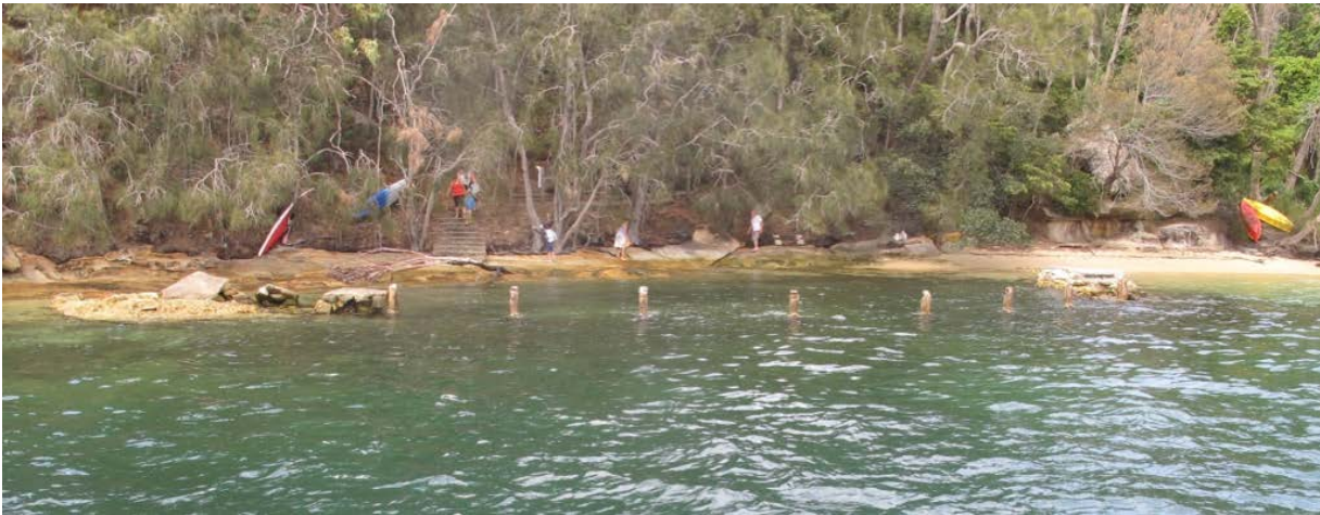
Figure 4-20: Clive Park Tidal Pool looking south towards shore. Row of eight reinforced concrete piles in the centre flanked by low sandstone walls bonded with cement. (Cosmos Archaeology 18 December 2017)
