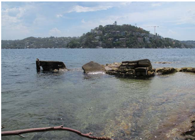
Figure 4-22: Eastern end of Clive Park Tidal Pool showing collapsed wall. Seaforth Bluff is in the background (Image: Cosmos Archaeology, 18 December 2017)
